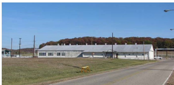
X-746 Shipping & Receiving Building
