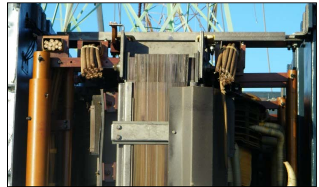
RIGHT: From the side, silicon steel that surrounds the copper core bundles is visible.
