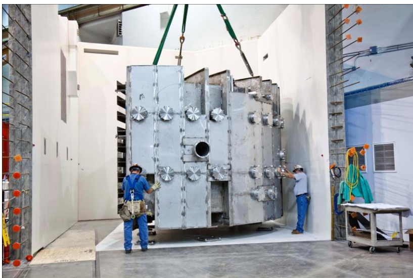
Fig. 5: Installation of the sample and detector tank of Corelli .
