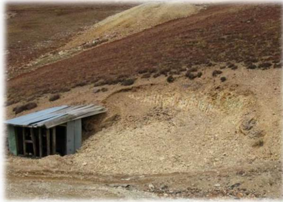
Number 1 Portal backfilled
