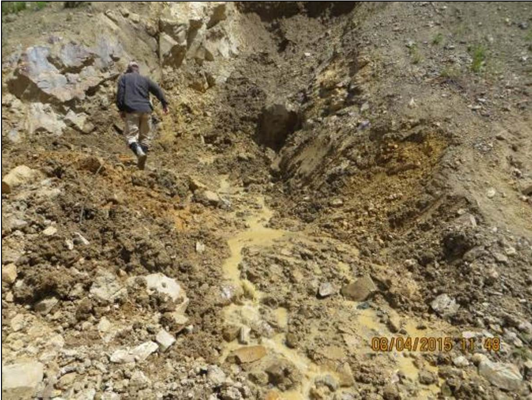
Figure 38.—Photograph showing seepage flow from the excavation at the Gold King Mine new portal at 11:48 a.m. on August 4, 2015. The flow is emerging approximately 5 to 6 feet above the floor of the adit (photograph from EPA project files).
