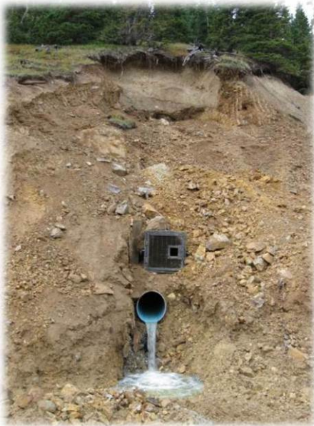
Gold King Level 7 Old Portal Closure
