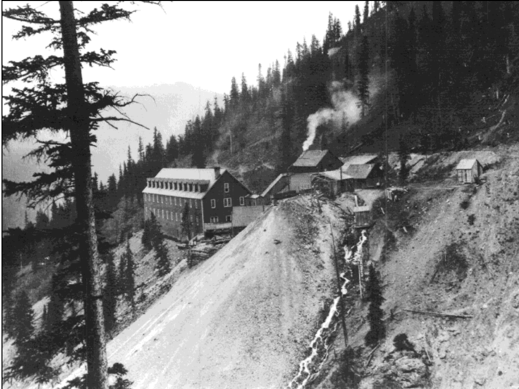
Figure 5.—Historical photograph of the Gold King Mine Level 7 taken prior to the mine closing in 1923. Note the drainage flow down the side of the waste-rock dump.
