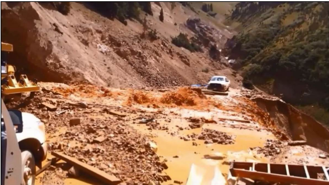
Figure 54.—Photograph showing the peak outflow from the blowout. The waste-rock dump is eroding on the right side of the photograph (still frame extracted from a video taken on August 5, 2015, at approximately 10:57 a.m.).
