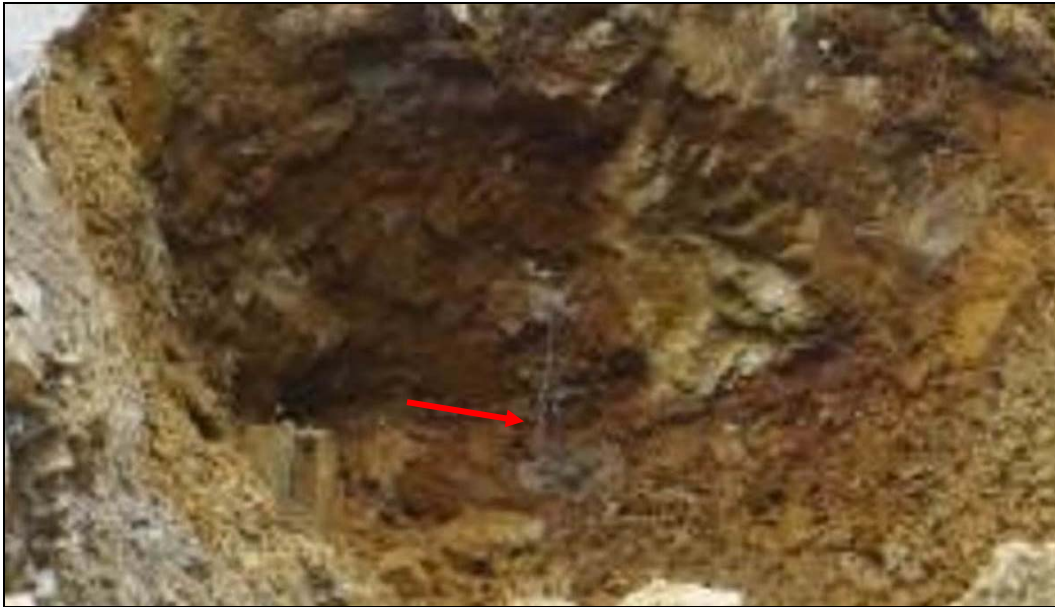
Figure 49.—A cropped and enlarged version of a portion of the photograph taken at 10:51 a.m. on August 5, 2015 (figure 48). Red arrow points to the initial vertical spurt of clear water shooting up about 1.5 to 2 feet as described by the EPA OSC (photograph from EPA project files).
