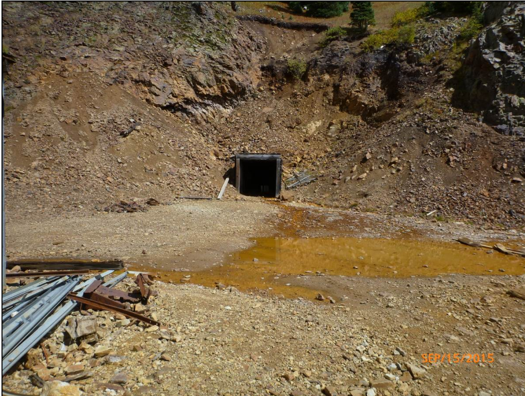
Figure 10.—Photograph showing seepage from the Mogul Mine on September 15, 2015. This mine has hydraulic bulkheads to limit the outflow of water from the Sunnyside Mine.
