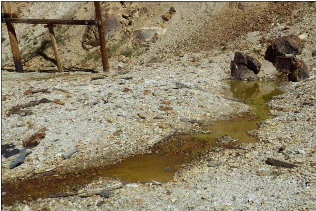
Figure 31.—Gold King Mine Level 7 OLD Adit (upper right) showing a small amount of seepage flow on September 11, 2014. At the portal, the floor of the old adit is approximately 2 feet higher than the floor of the old adit portal (photograph from EPA project files).
