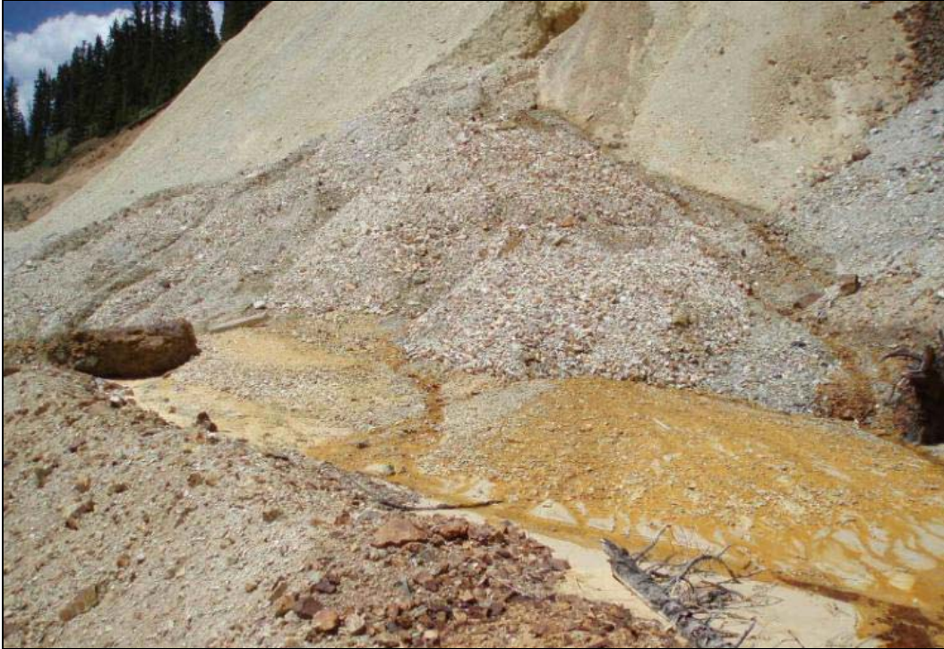
Figure 15.—Photograph showing deposition of landslide material in 2007 blocking a portion of the access road near the base of the waste-rock dump (from DRMS project files).
