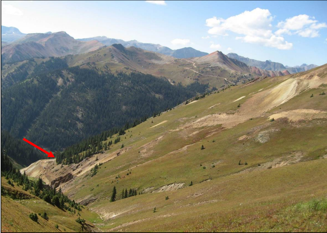
Figure 1.—Photograph of the Gold King Mine looking west. The red arrow points to the location of the mine blowout, which occurred on August 5, 2015.
