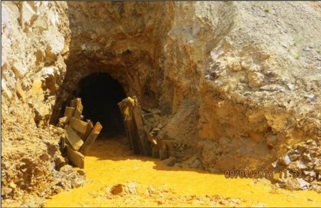
Figure 59.—Photograph showing the condition of the adit at 11:33 a.m., August 5, 2015; the peak flow of the uncontrolled release had passed and the flow rate was decreasing (photograph from EPA project files).
