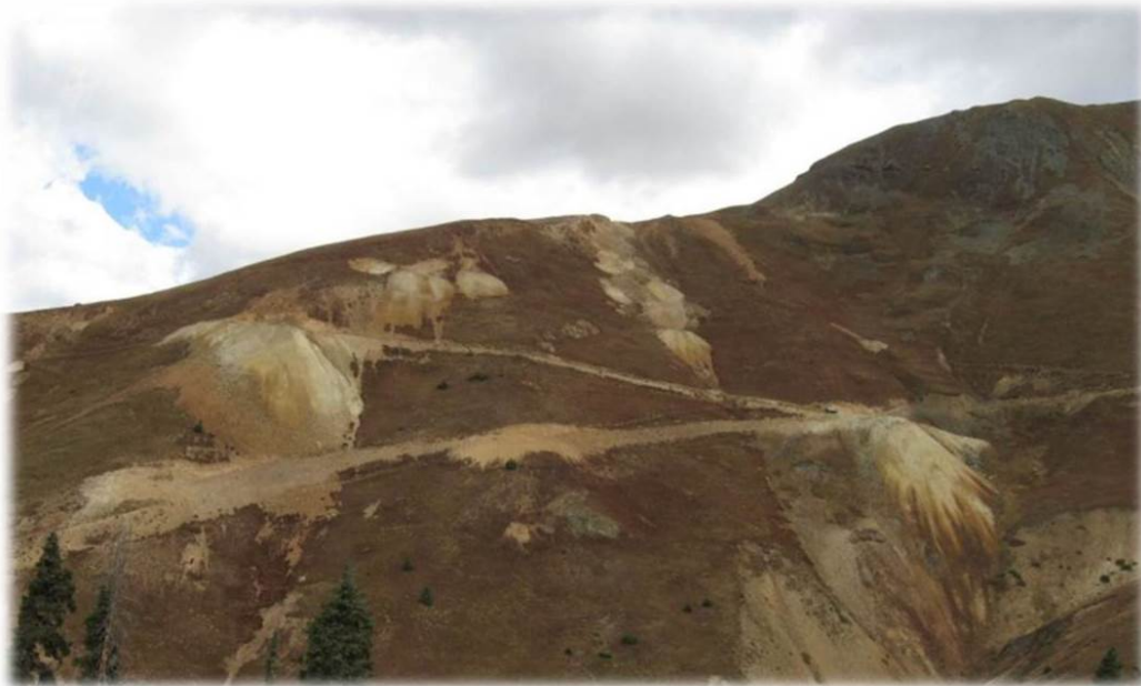
Sampson Portal, Drill Road, and Number 1 Portal as viewed from access road after reclamation. Drill Road has been re-contoured and revegetated in this photo.
