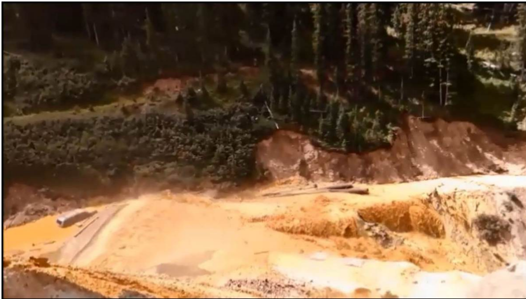
Figure 56.—Photograph showing at left, the inundation of a vehicle parked near the base of the waste-rock dump, and on the right water overwhelming the access road and cascading down into the North Fork of Cement Creek (still frame extracted from a video taken on August 5, 2015, at approximately 10:57 a.m.).
