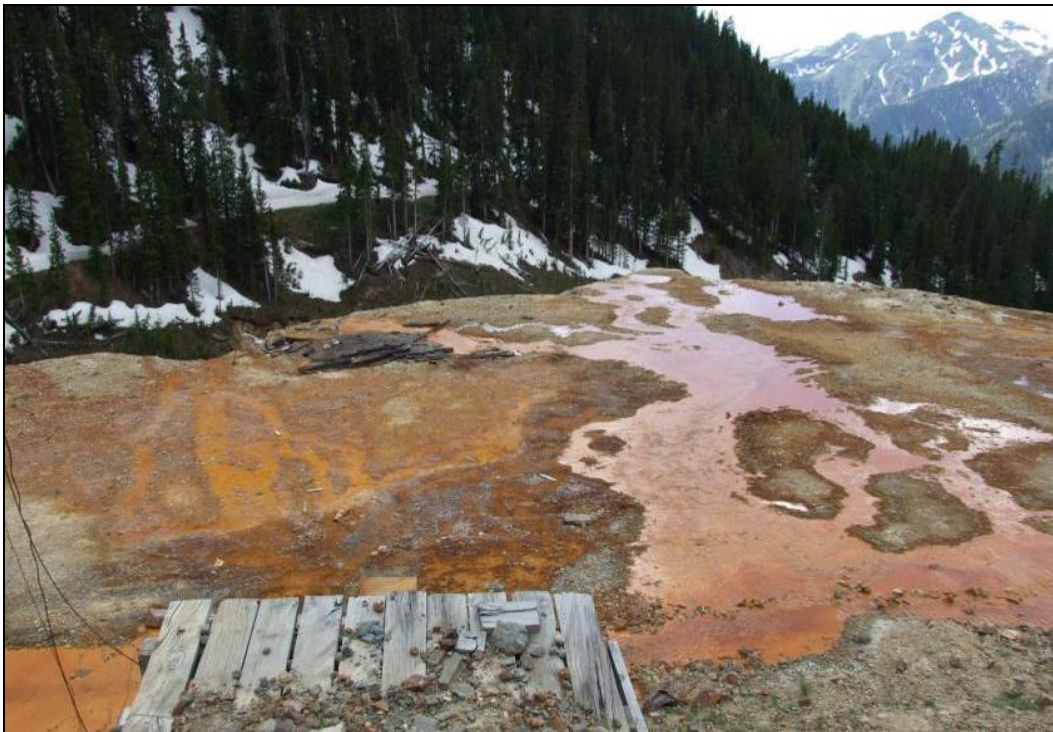
Figure 14.—Photograph showing adit seepage infiltrating into the Gold King Mine Level 7 waste-rock dump in 2007 (from DRMS project files).
