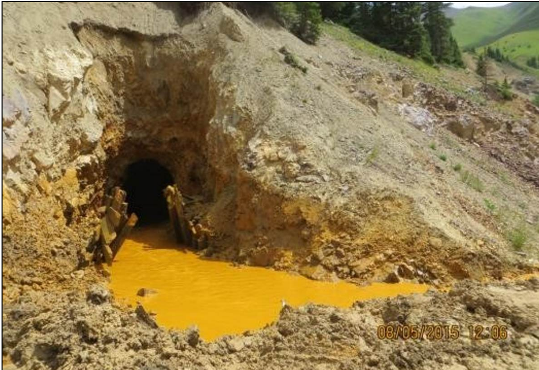
Figure 60.—Photograph showing that the flow had been routed back toward the half-round pipe by 12:06 p.m. on August 5, 2015 (photograph from EPA Project Files).
