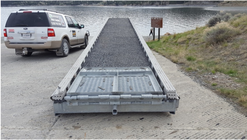
Figure 7: Shannon Recreation Area Courtesy Boat Dock. Image is taken after the incident. Access Ramp is in a fully closed position, folded onto the surface of the Dock. Image courtesy of the Lewis and Clark County Sheriff's Department.
