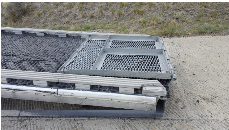
Figure 2: Access Ramp, folded closed onto the Dock.
