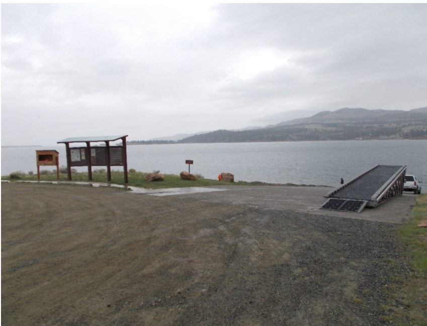
Figure 6: Shannon Recreation Area Courtesy Boat Dock. Image is taken after the incident. Access Ramp is in a fully open position in contact with the ground. Image courtesy of the Lewis and Clark County Sheriff's Department.
