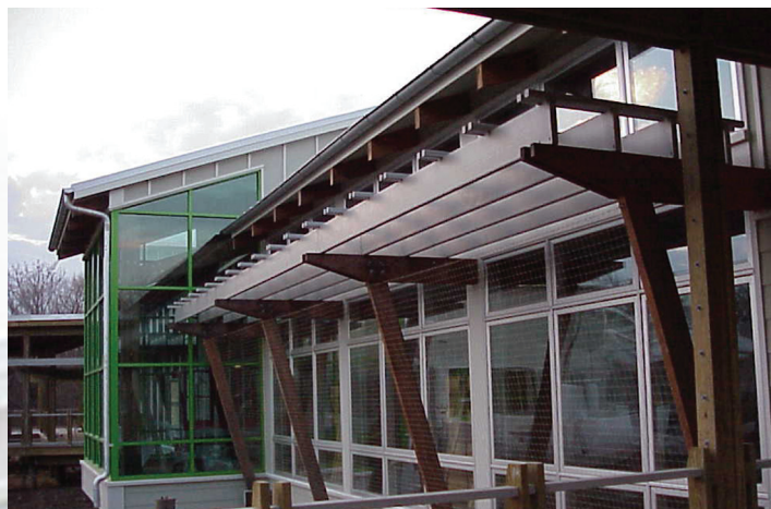
Bird Collision Netting at the Cusano Environmental Education Center, John Heinz NWR at Tinicum, Pennsylvania. Photo credit: US Fish and Wildlife Service
