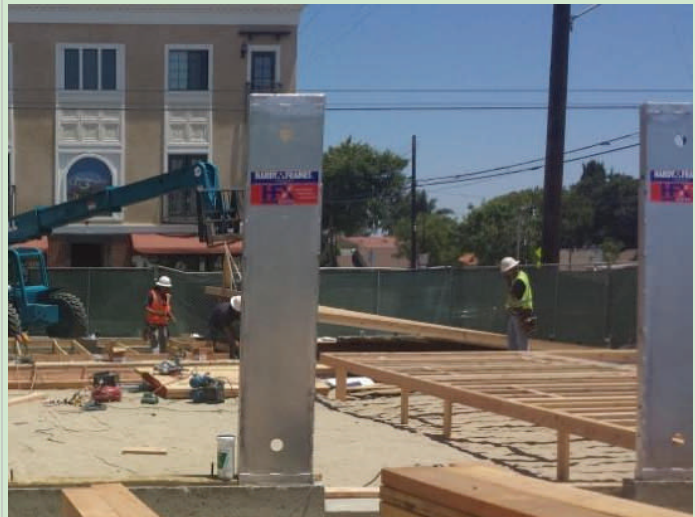
View of new construction at Café Camellia/Fronk's Restaurant Site.
