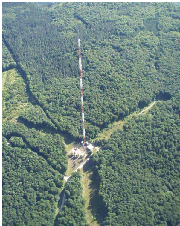
Figure 5. Seven communication towers located throughout the lower Peninsula of Michigan were included in a study of avian collisions (six each season). The areas under these towers were simultaneously and systematically searched for bird carcasses during 20 consecutive mornings surrounding the peak of songbird migration in the spring and fall 2008 and 2009 to compare the relationships between avian fatalities and tower lighting systems.
