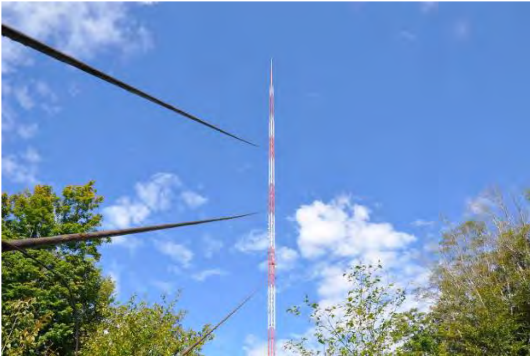
Figure 3. Guy Wires Supporting the WPBN Tower
