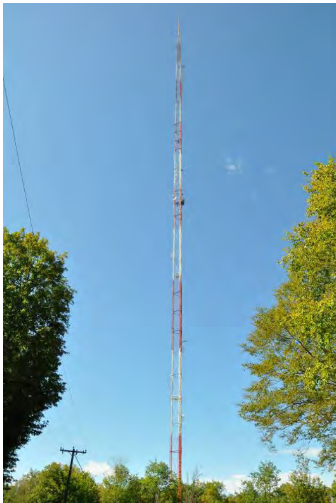
Figure 1. The WPBN Tower, Harrietta, Michigan
