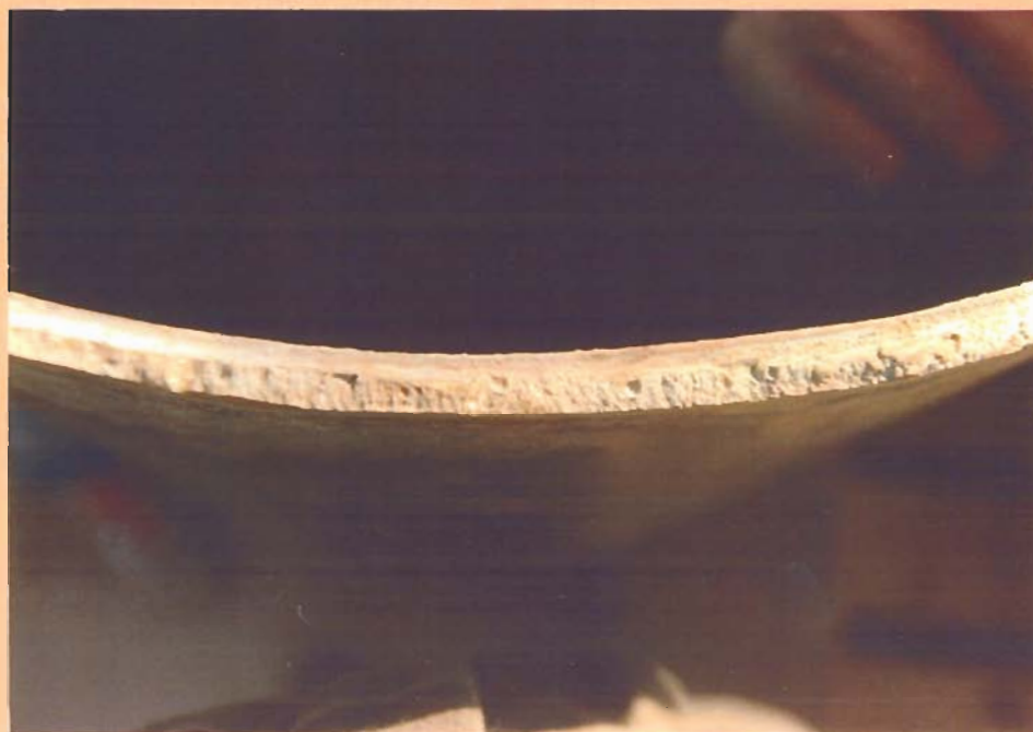
Figure 2 Lack of Penetration in Circumferential Weld
