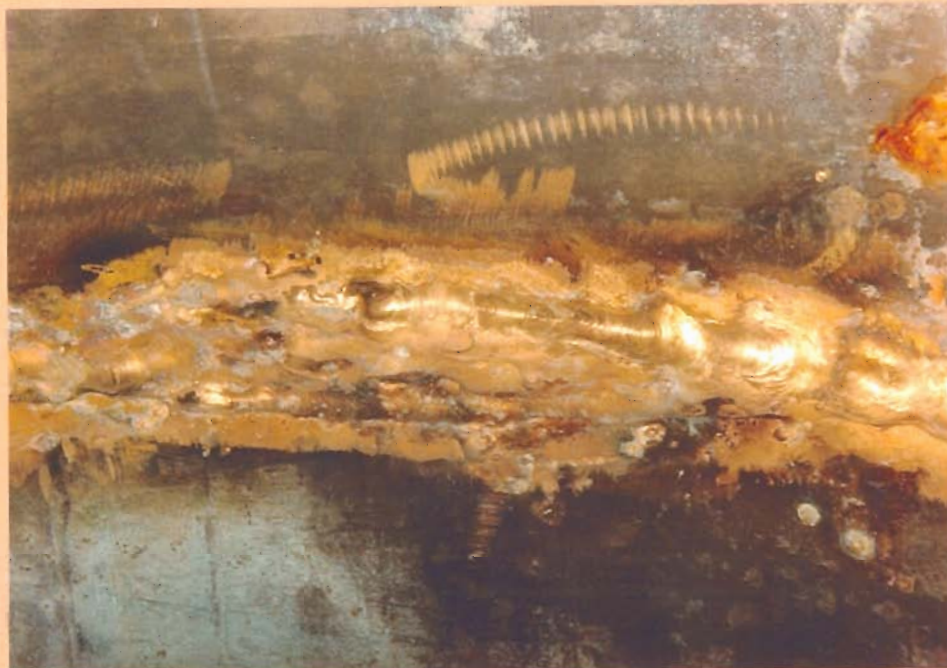
Figure 1 Surface Appearance of Repaired Circumferential Weld
