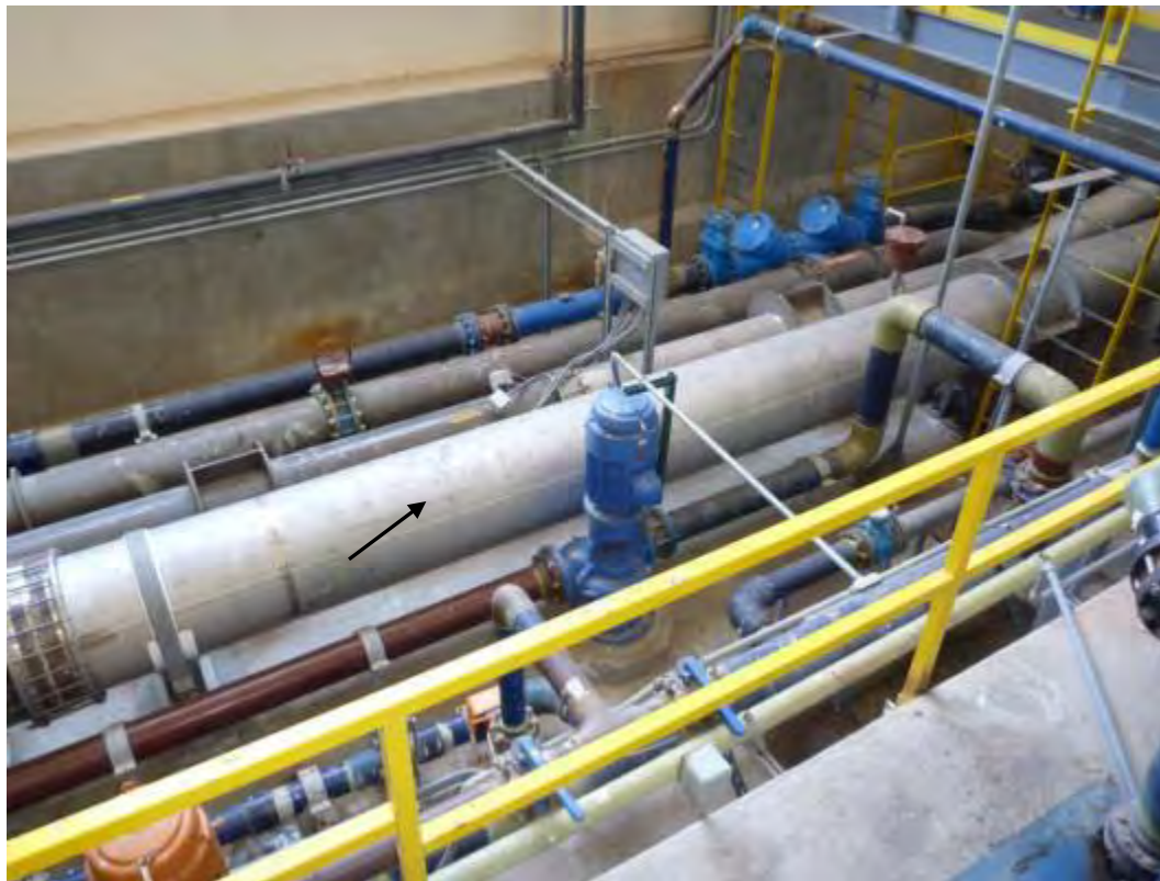
Photograph 7. A replaced segment of concentrate piping.
