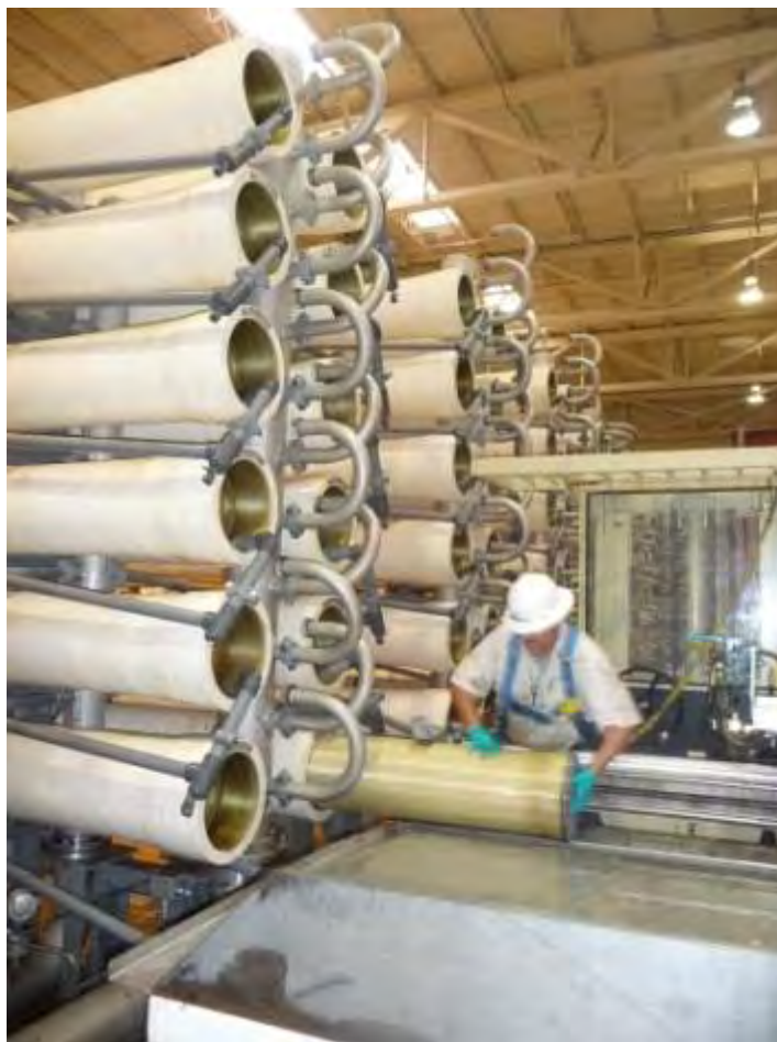
Photograph 11. Loading one of 2,304 membranes.
