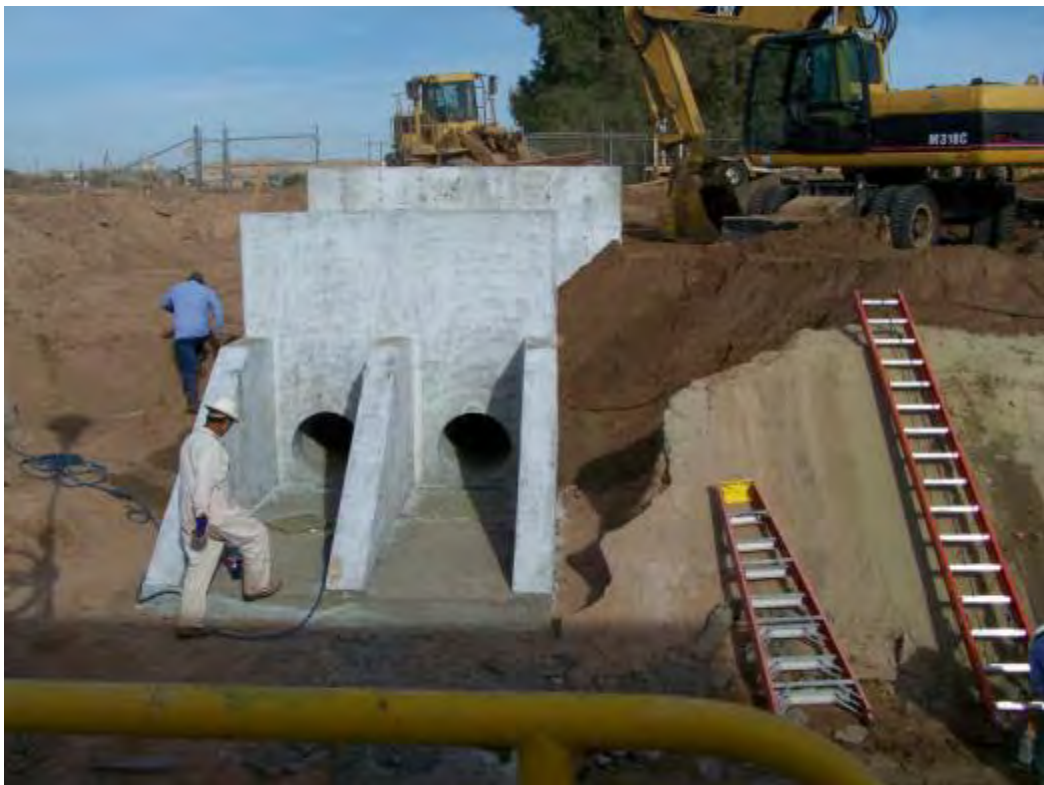
Photograph 9. New MODE 2 blend flow system under construction.
