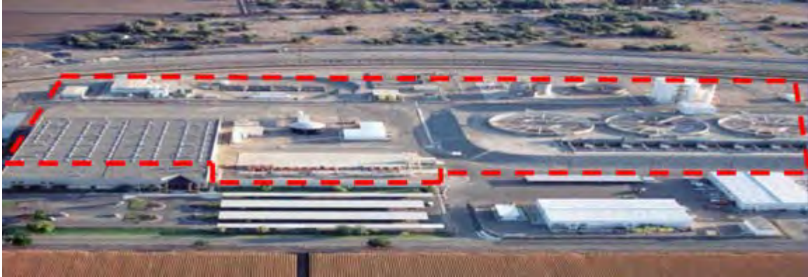
Photograph 10. YDP Controlled Access Zone.
