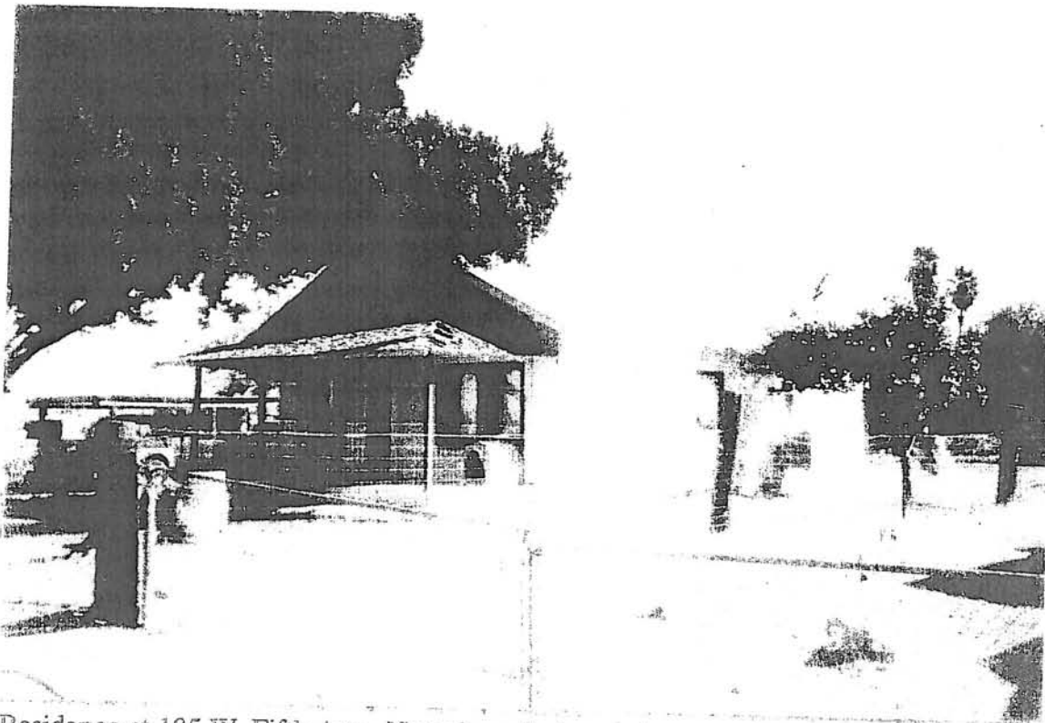
Residence at 185 W. Fifth Ave. Note the rolled asphalt on south-facing portion of roof.
