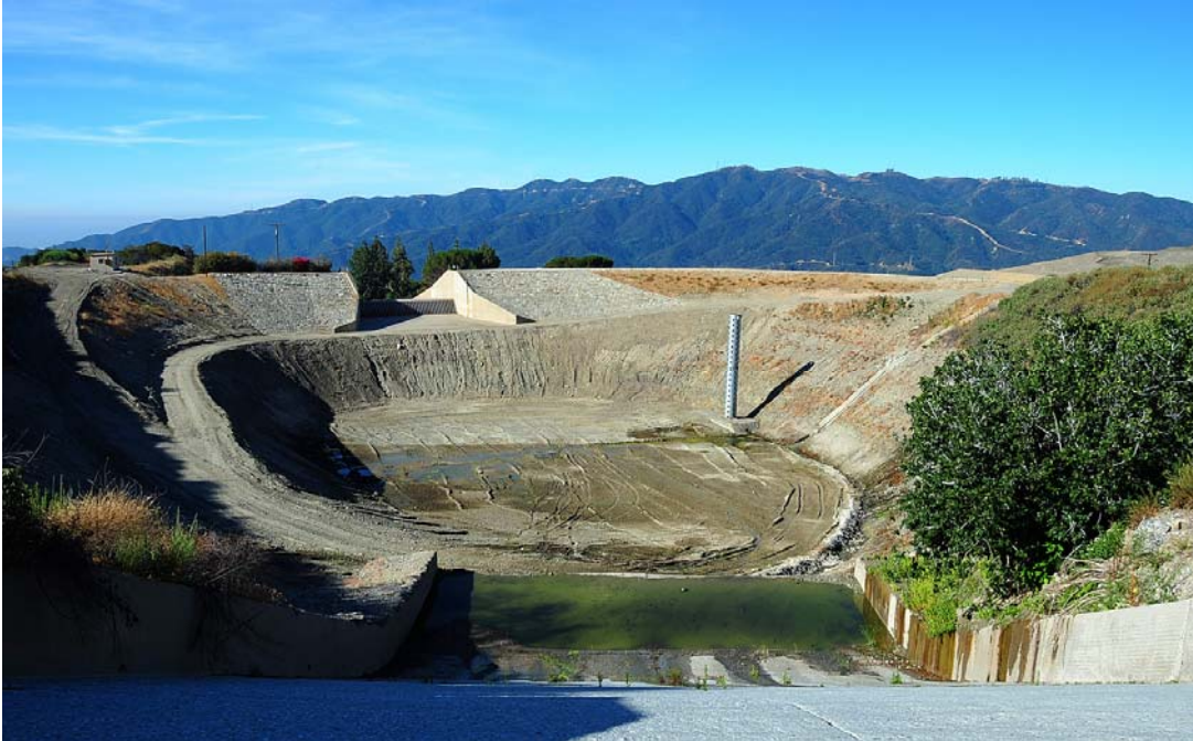
Photo 18. Dunsmuir Debris Basin, Los Angeles County, California.
