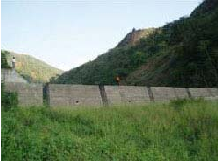
Photo 15. Slit-type check dam in Vargas Province, Venezuela Source: http://www.sabo-int.org/projects/venezuela.html
