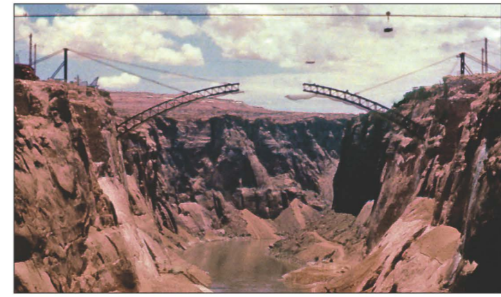
Colorado River Bridge construction, February, 1958
