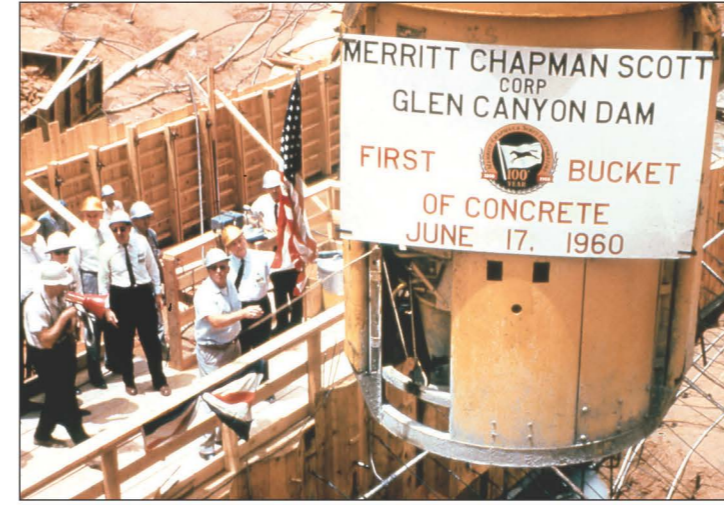
First bucket of concrete
