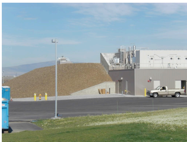
Figure 22 – Surface berm of Building 3425 in July 2010 at completion of construction. Note additional rock cap earthen bunker compared to Figure 21.
