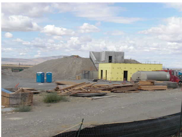
Figure 21 – Surface earthen berm from southeast of Building 3425 in August 2009 during construction.
