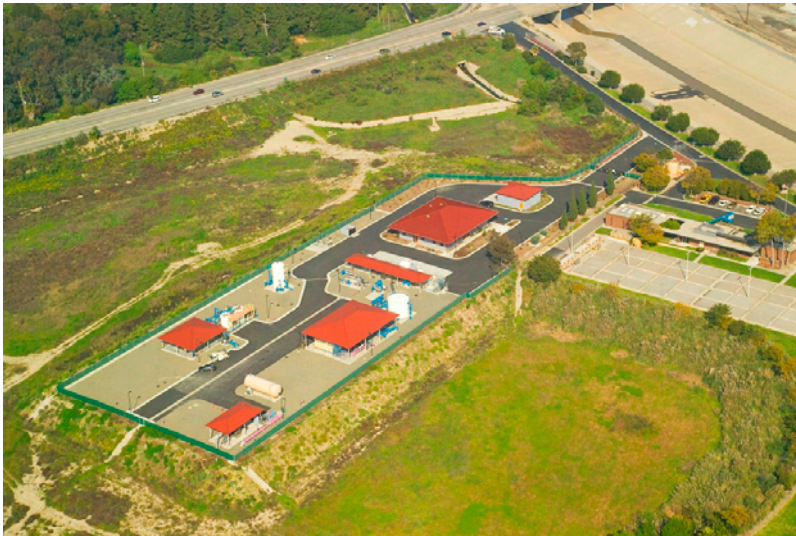
FIGURE 8.1 AERIAL OF LEO VANDER LANS ADVANCED WATER TREATMENT FACILITY
