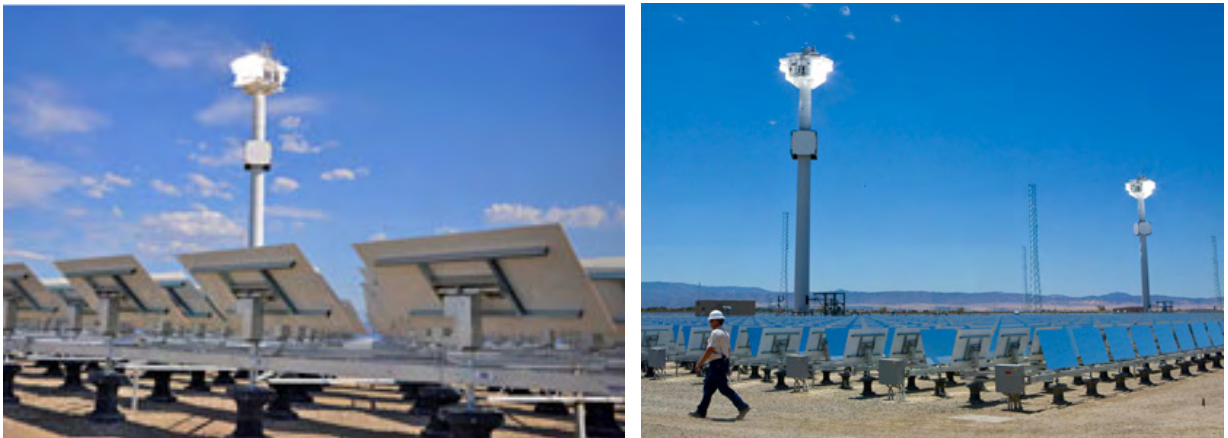
FIGURE 13.1 SIERRA SUNTOWER POWER PLANT
