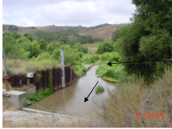
Figure 5. Looking across from left bank at O'Neill Diversion Weir and majority of river flow shown in Figure 4 being diverted into canal.
