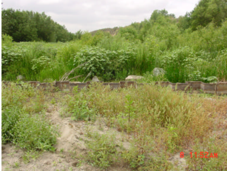
Figure 6. Looking downstream along middle of channel at sediment piled up against existing sheet-pile diversion weir (6-8-2004).
