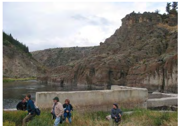
Photo 2-24. View looking west from Linderman Dam reveals the old concrete dam structure in the foreground, small pool and rugged cliffs in the middleground, and steep, disturbed cliffs in the background.
