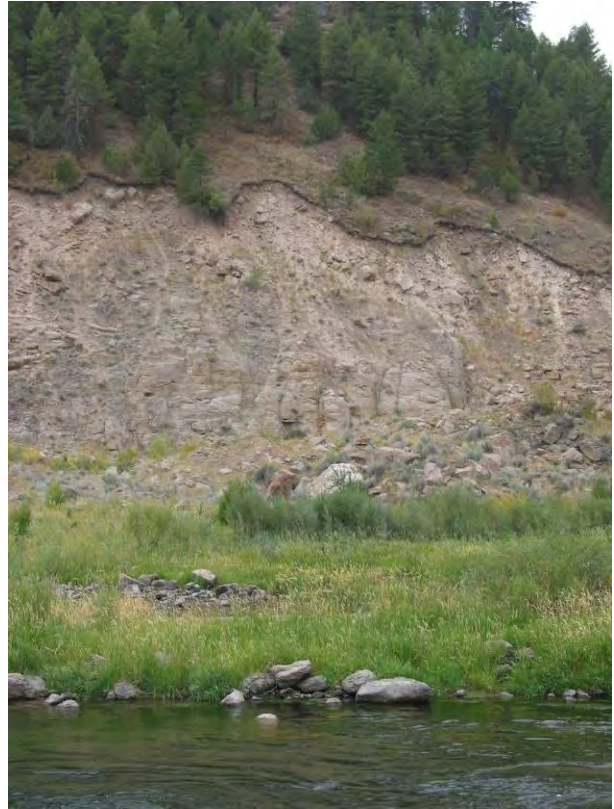
Photo 2-4. Typical view from the canyon floor of a slide and source material below.
