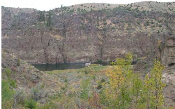
Photo 2-22. View looking north from the Linderman Dam Access trail reveals the flat canyon bottom in the foreground, old concrete dam structure and river in the middleground, and steep, rugged cliffs in the background.
