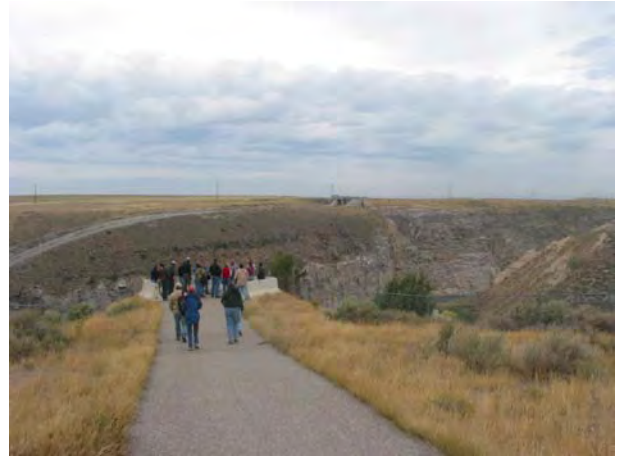
Photo 3-4. Teton Dam Overlook with the spillway seen in the background.
