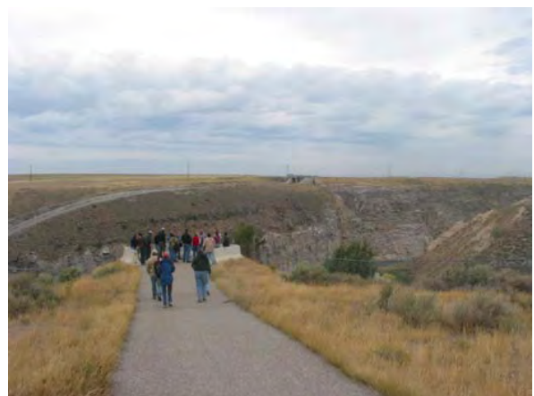
Photo 2-16. Approach to the Teton Dam Overlook with the old spillway and dam in the background.
