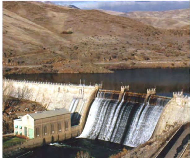
Photo 1-2. Black Canyon Dam and adjacent powerplant.
