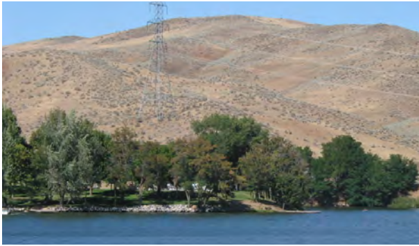
Photo 2-4. Riprap along the south side of Black Canyon Park.
