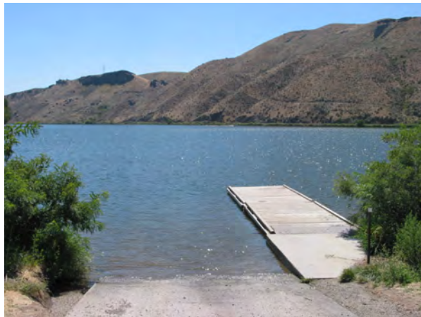
Photo 3-16. Highway County Boat Ramp #1.
