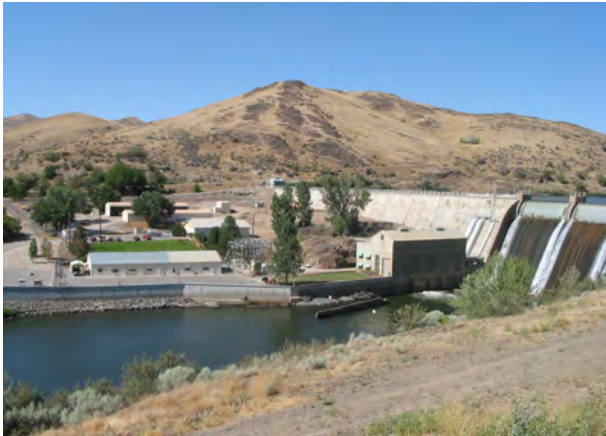
Photo 3-1. Black Canyon Dam, powerhouse, and operations facility.
