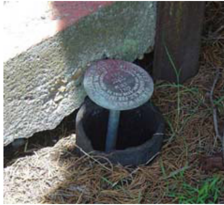
The position of this vertical survey marker in Louisiana has been upset due to significant subsidence (sinking) of the surrounding area. Click on the image for a larger view.
