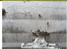
Possible Lead Based Paint
