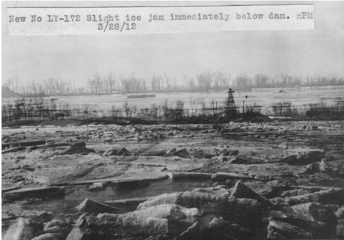
Figure A5. Jam below the Intake Dam at the onset of the March 28, 1912 breakup.
