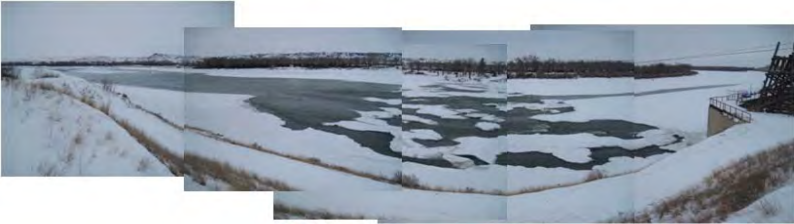
Figure A1. View of Intake Dam from the north on January 14, 2011. Flow is right to left.
