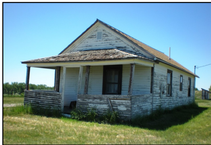
Figure 4-3. Headworks gate tender's residence
