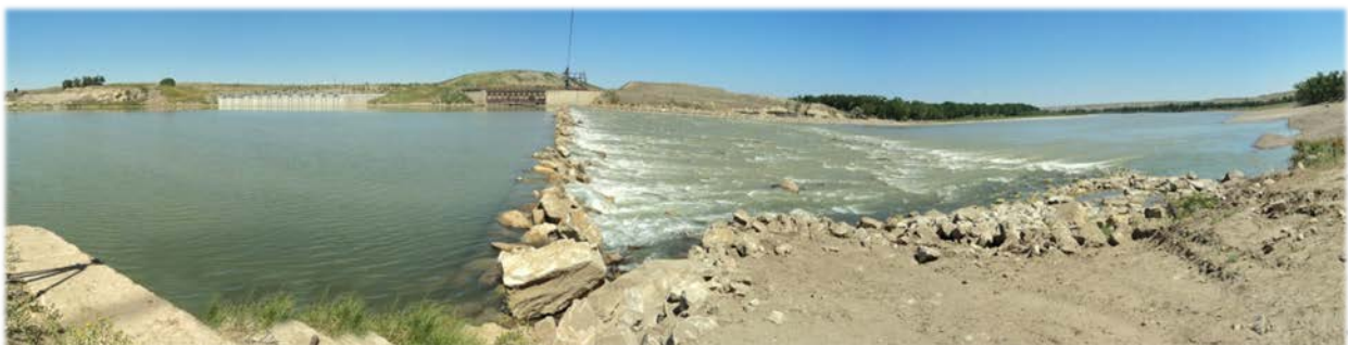
Photograph 22 - View of Intake Dam from right descending bank of the Yellowstone River facing north
