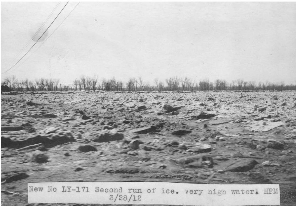
Figure A6. Second ice run during March 28, 1912.
