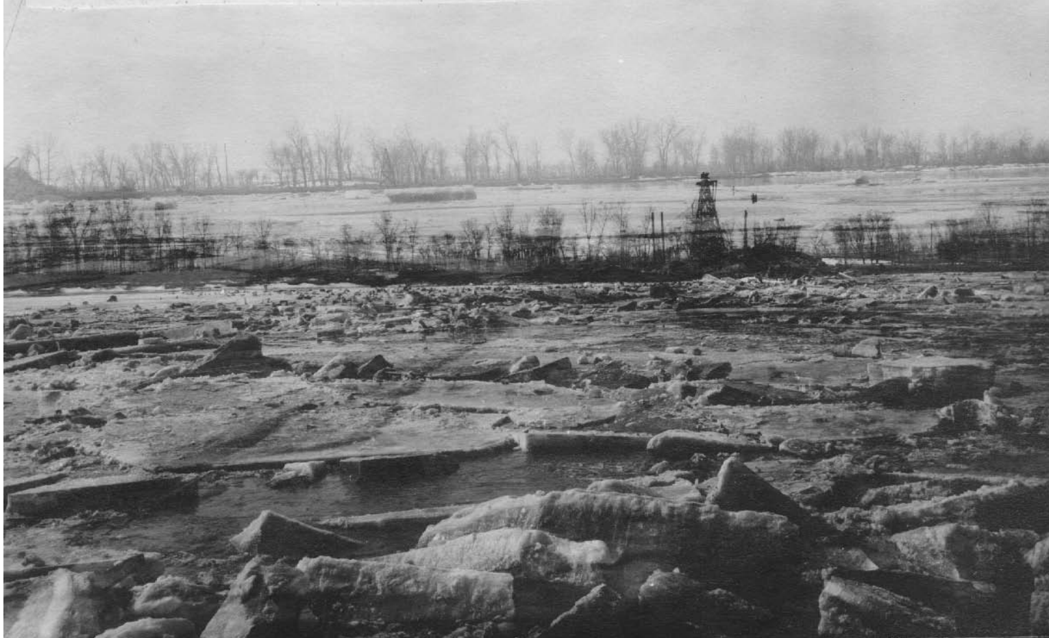
Fig. 3. Ice jam on the Yellowstone River at the Intake in 1912 forcing flow and ice into the right overbank area.
