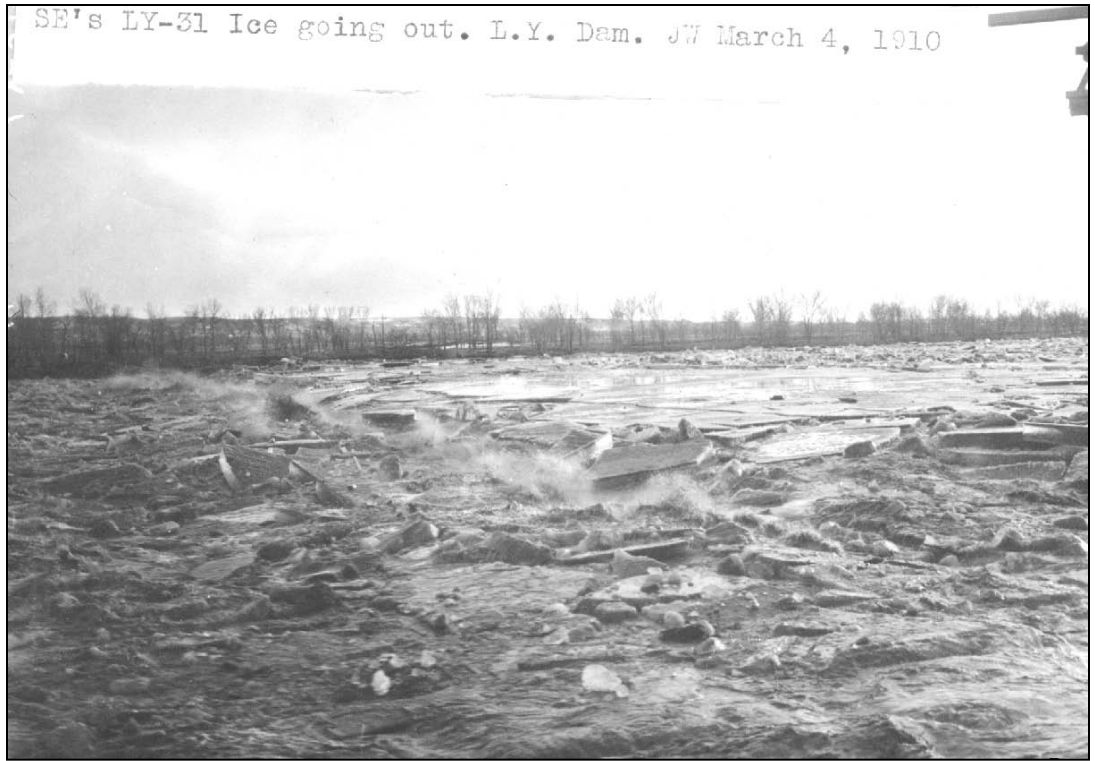
Figure A3. Ice moving over the newly completed dam on March 4, 1910.
