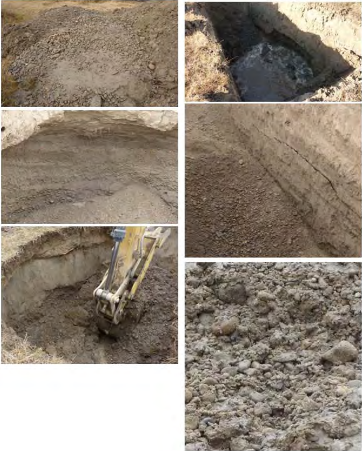
Figure 7 - Bypass Test Pit Photos
