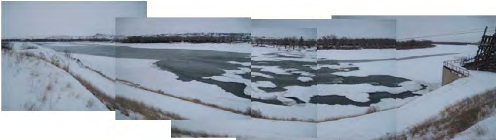
Figure A1. View of Intake Dam from the north on January 14, 2011. Flow is right to left.
