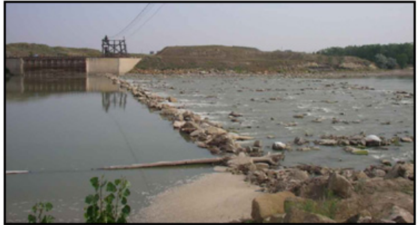
Intake Diversion Dam
