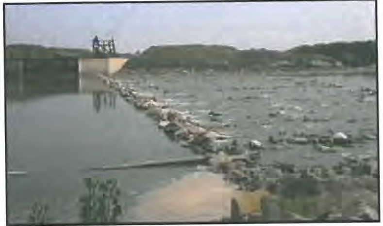
Intake Diversion Dam
