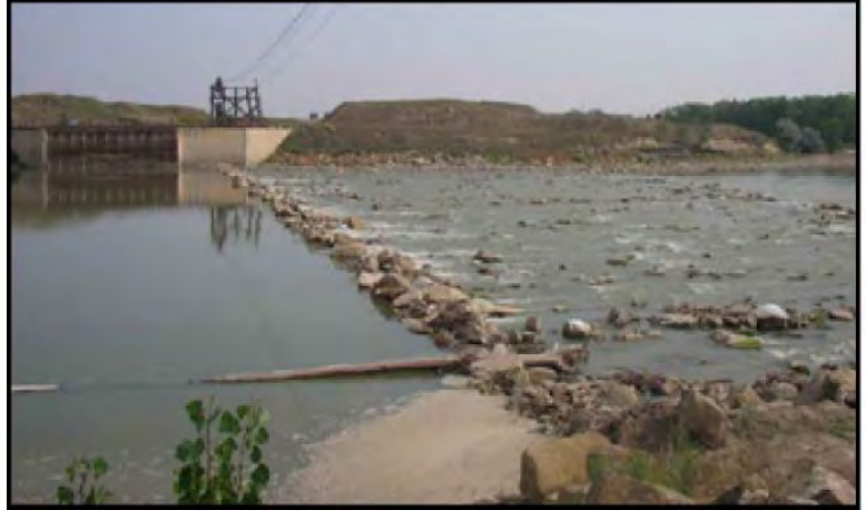
Intake Diversion Dam
