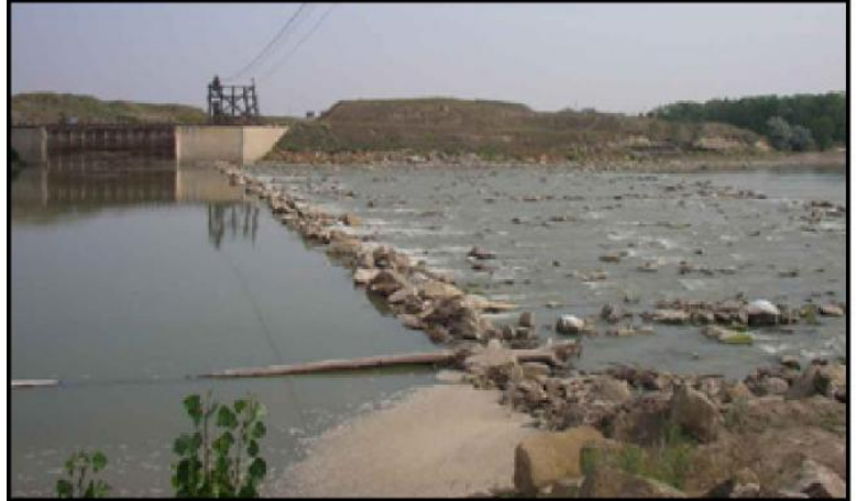
Intake Diversion Dam
