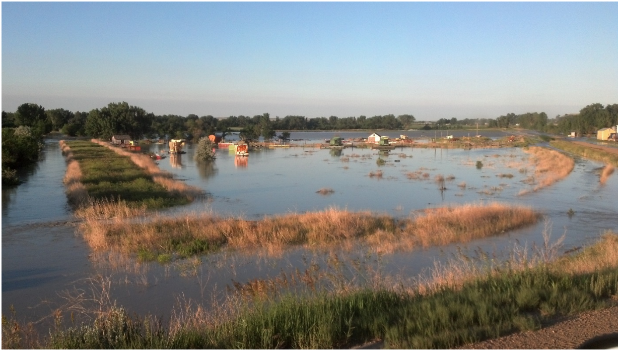
Main Canal – Photo of Small Washout (LYIP 2012)
