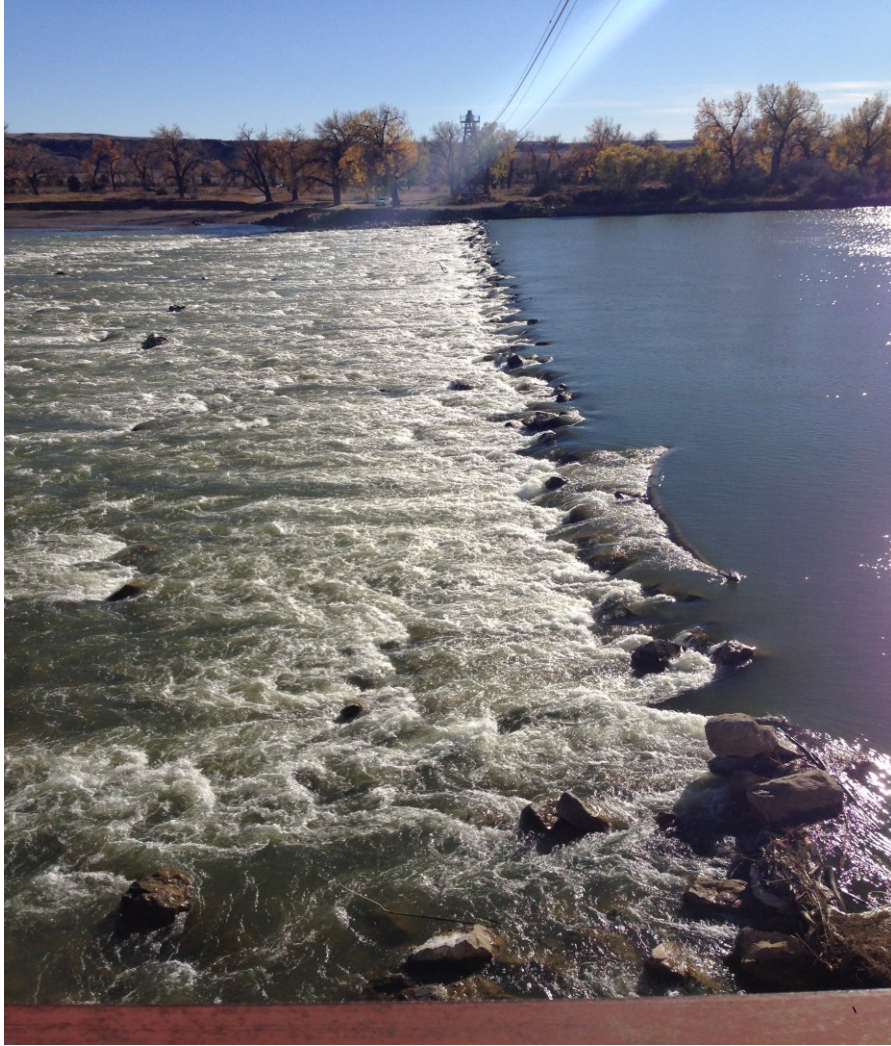
Figure 3-7. Intake Diversion Dam
