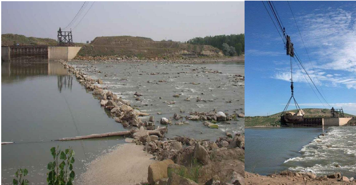
Figure 3-24. (Left) Low Water Exposes the Intake Diversion Dam Rock Weir; (Right) Higher Waters Create Riffle, Overhead Cableway Delivers Rocks to Weir
