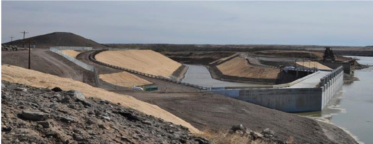
Figure 3-25. New Headworks at the Entrance of the Main Canal with Fish Screens Completed in 2011
