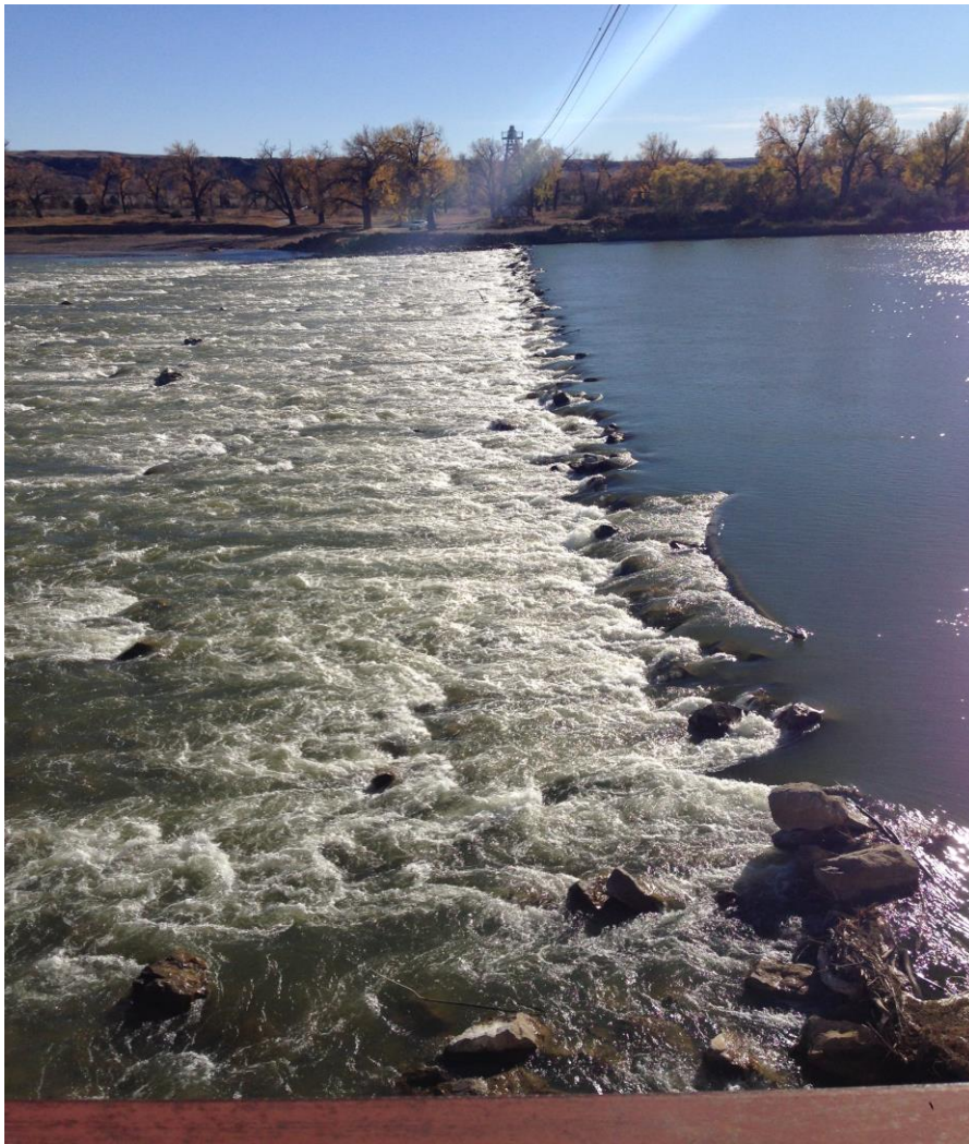
Figure 3-7. Intake Diversion Dam
