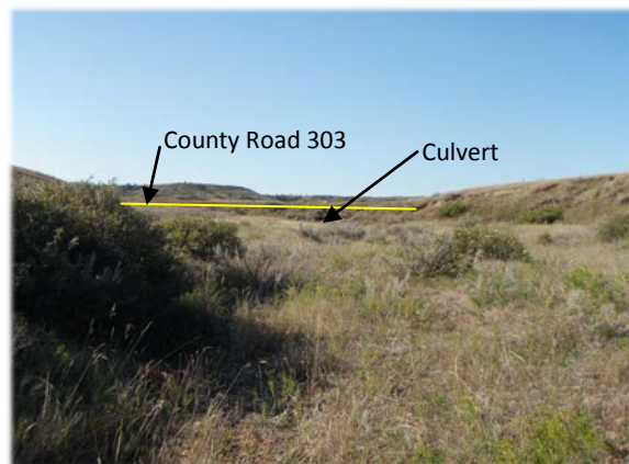
Photograph 2 – View from west of PS-1 from within DW-1 facing upstream
