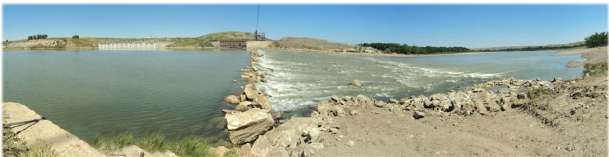
Photograph 22 - View of Intake Dam from right descending bank of the Yellowstone River facing north
