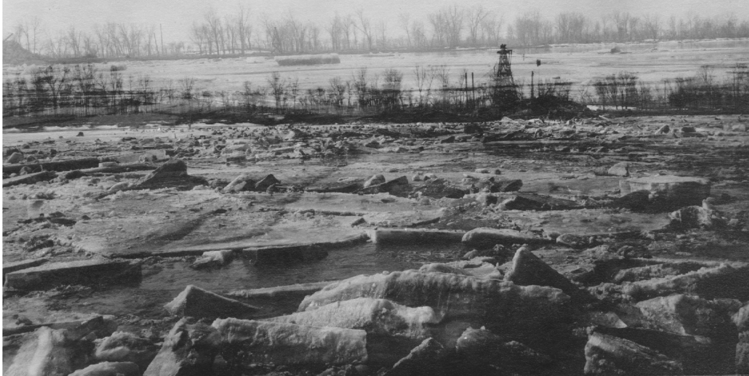
Fig. 3. Ice jam on the Yellowstone River at the Intake in 1912 forcing flow and ice into the right overbank area.
