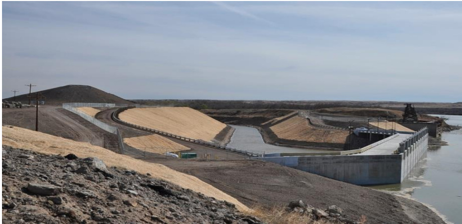
Figure 1 - New Headworks with Fish Screen at Intake (screens submerged)
