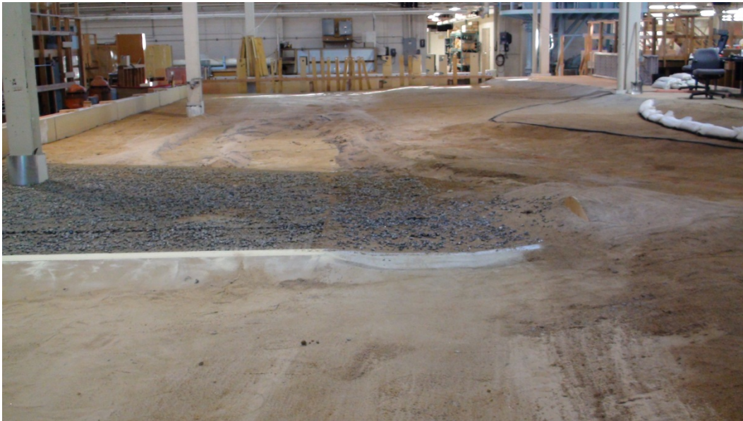
Figure 17. Low flow notch on right side of diversion weir.
