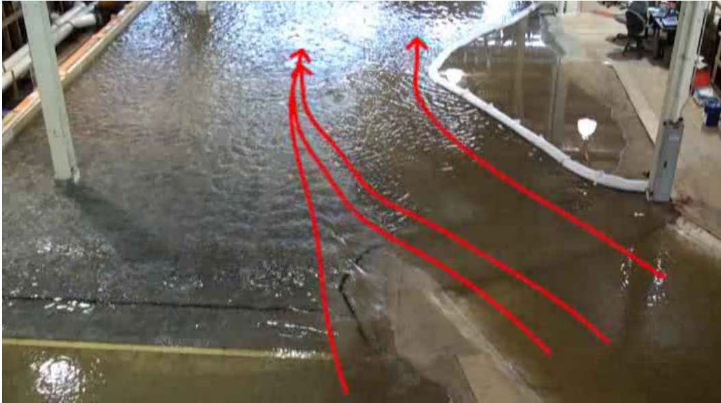
Figure 15. Fish bypass entrance flow patterns, configuration 4 (bypass invert 1981 ft, right bank topography adjustment- large, center point topography adjustment), total river flow= 45,300 ft 3 /s
