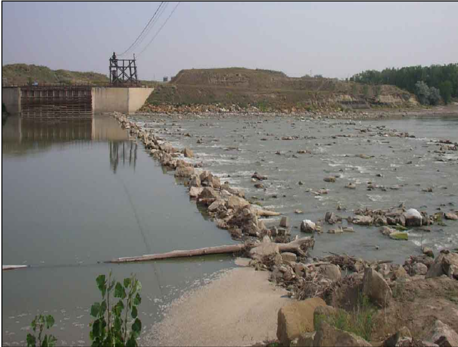
Figure 2: Existing Diversion Structure
