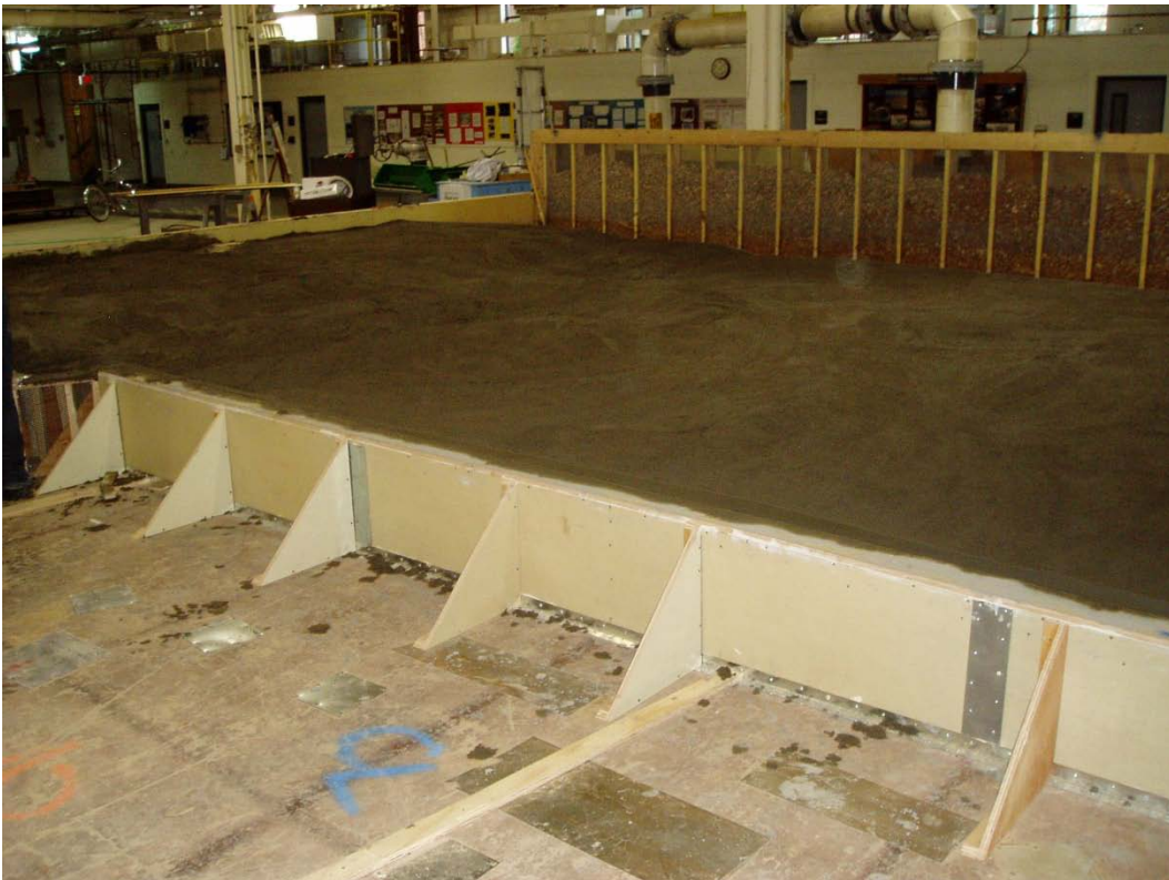
Figure D- 3. Concrete layer over upstream topography.
