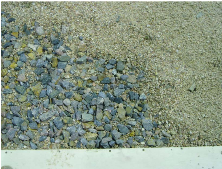
Figure 15. Photo showing the rock ramp with washed choke material in the bottom left corner and the choking layer prior to washing into the rock in the top right corner.
