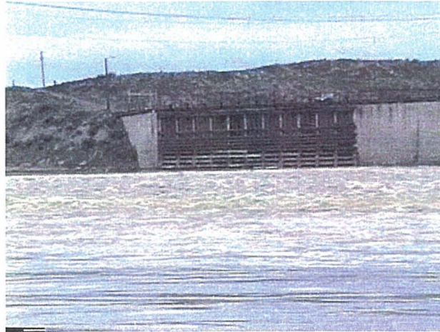
Figure 2 - View of Intake Dam and Main Canal Headworks.
