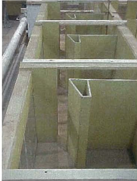
View of standard vertical slot baffle fishway looking downstream.
