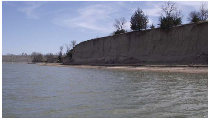
Location of additional 50' breakwater, referenced as Location #1.
