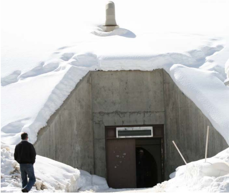
Figure 17. Photograph of the LMDT portal structure taken on March 25, 2008.
