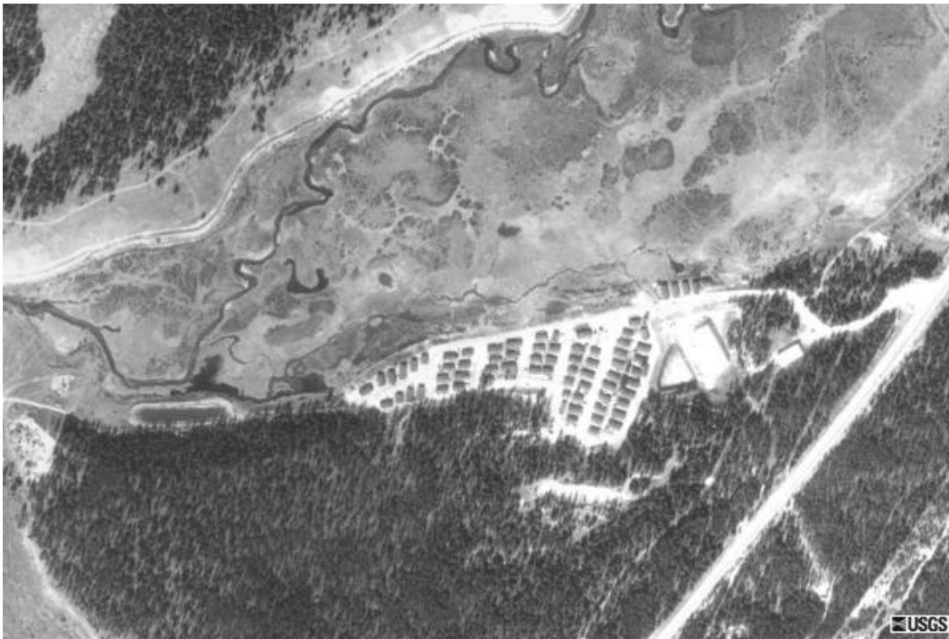
Figure 27. Aerial Photograph Showing the LMDT Portal Area Including the Water Treatment Plant, Adjacent Housing, and East Fork of the Arkansas River.
