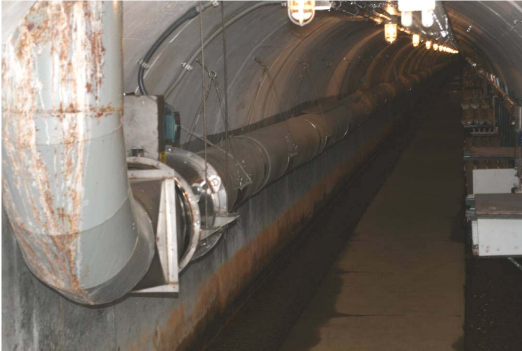
Figure 19. Photograph taken on March 25, 2008 looking upstream from the Portal area in the LMDT showing the ventilation fan, motor controls, and vent pipe at left, and the electric lights at the upper right.
