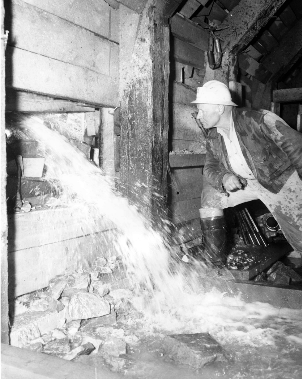
Figure 12. Photograph showing the inflow to the LMDT through a drillhole connected to the Robert Emmet shaft, taken from (Salsbury, 1956). This is prior to driving the Robert Emmet lateral.
