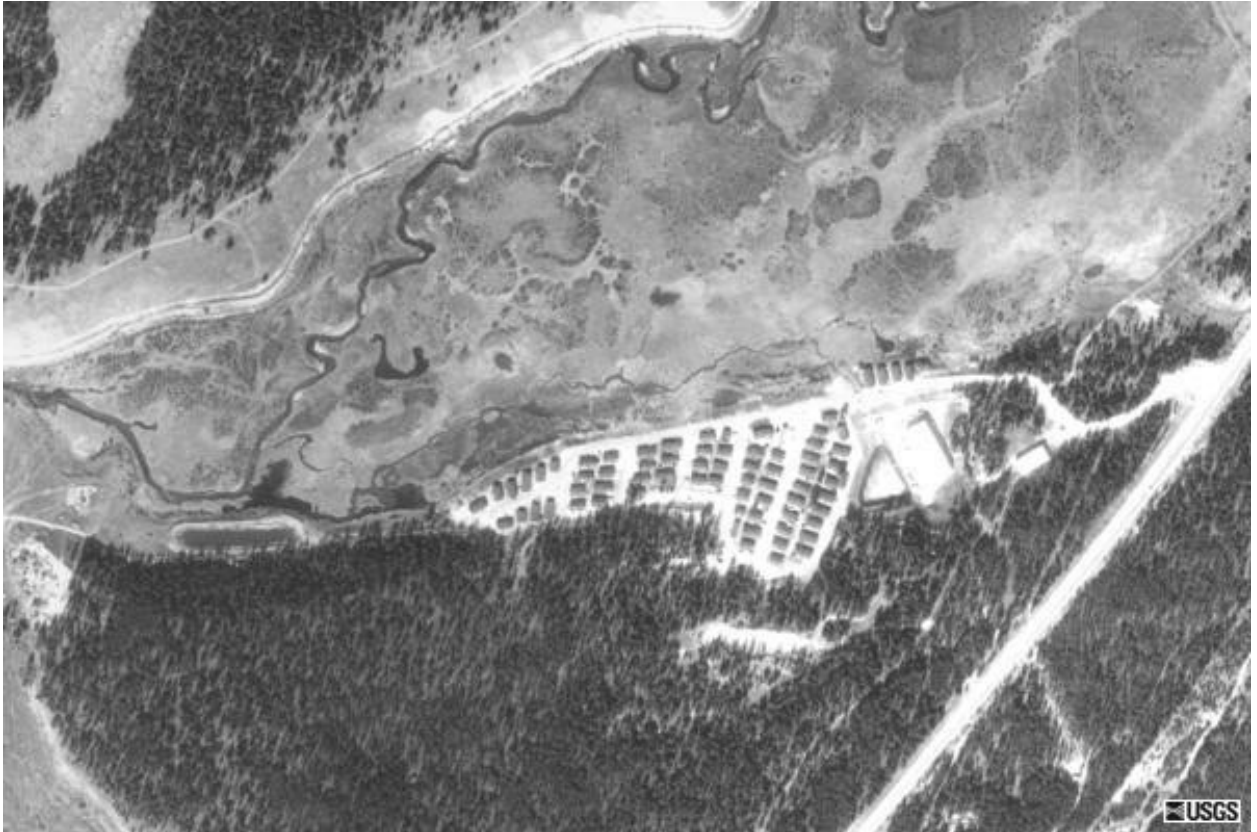
Figure 7. Recent Aerial View of Tunnel Portal Area
