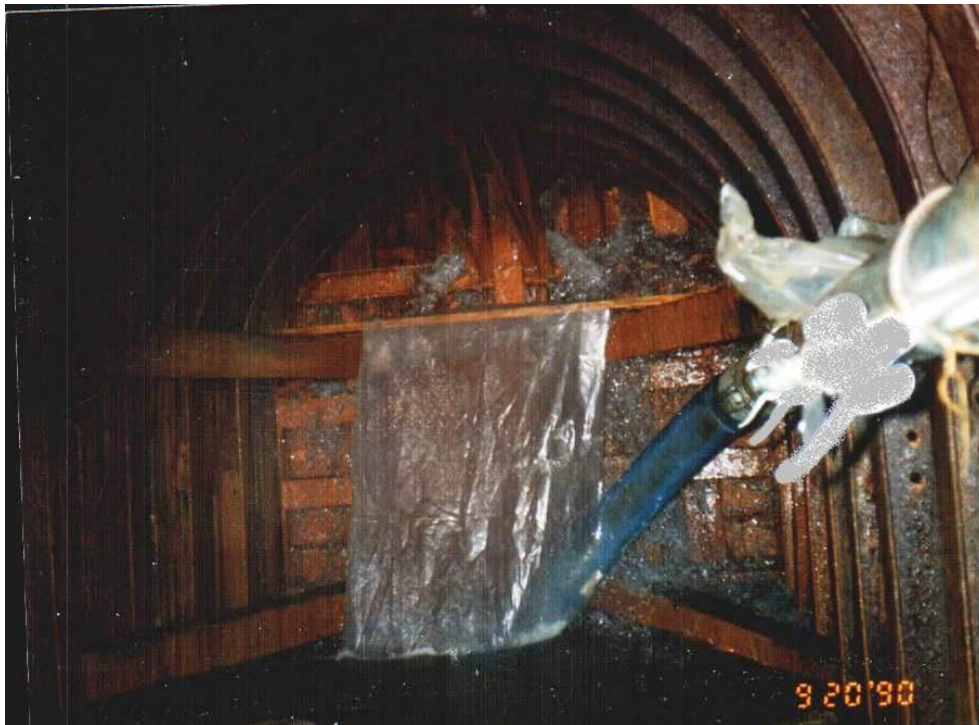
Figure 15. Photograph of the bulkhead located at Station 4+66.
