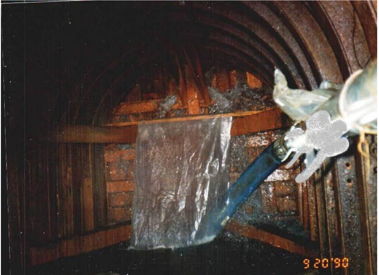
Figure 6. Bulkhead at Station 4+66 (date noted on photo)
