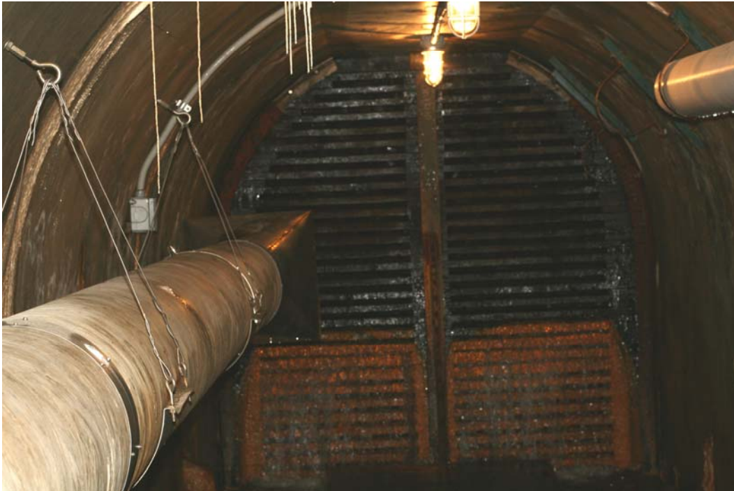
Figure 23. Photograph taken on March 25, 2008 of the cobble and gravel-filled timber-lattice bulkhead at Station 4+61 of the LMDT. At left is the intake end of the ventilation pipeline.
