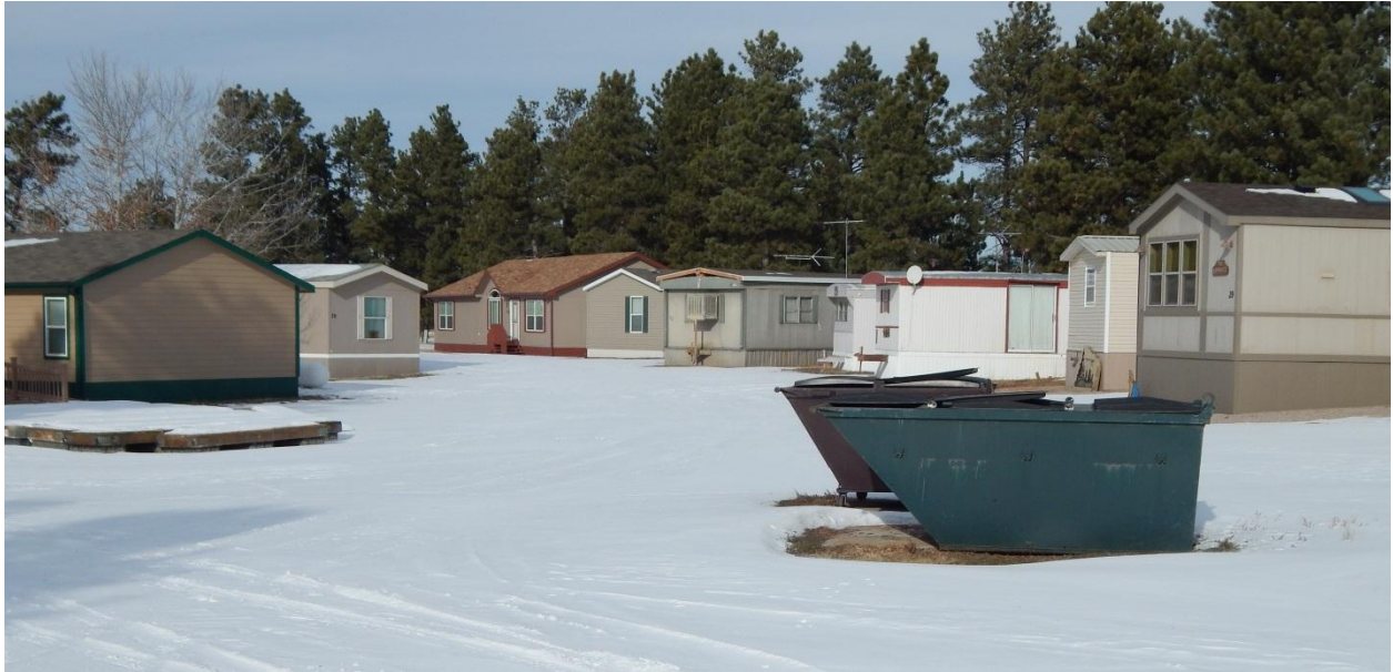
From left to right, the mobile homes on Trailer Sites 40, 39, 35, 34, 33, 32, 31, 30, and 29.
