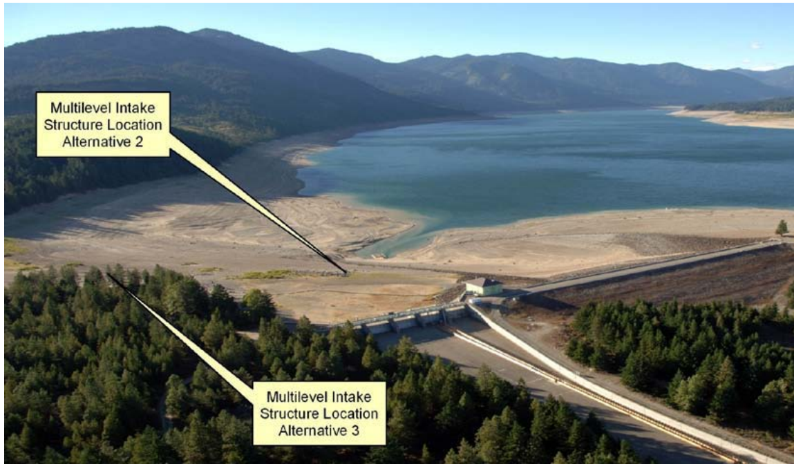
Figure 4-11. Aerial view of Cle Elum Dam showing approximate locations of intake structures for both action alternatives. Pool elevation is 2,119 feet in this photo
