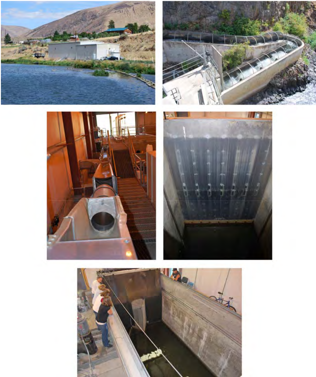
Figure 2-3. View of exterior of Roza adult fish collection facility (top left); pool and weir-type fish ladder (top right); fish chute to work area or back to river (middle left); fish lock (middle right); and adult holding tank (bottom, right).
