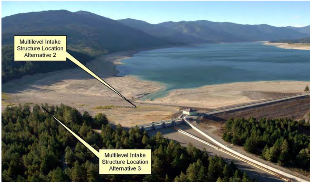
Figure 2-7. Aerial view of Cle Elum Dam showing approximate locations of intake structures for both action alternatives. Pool elevation is 2,119 feet in this photo.
