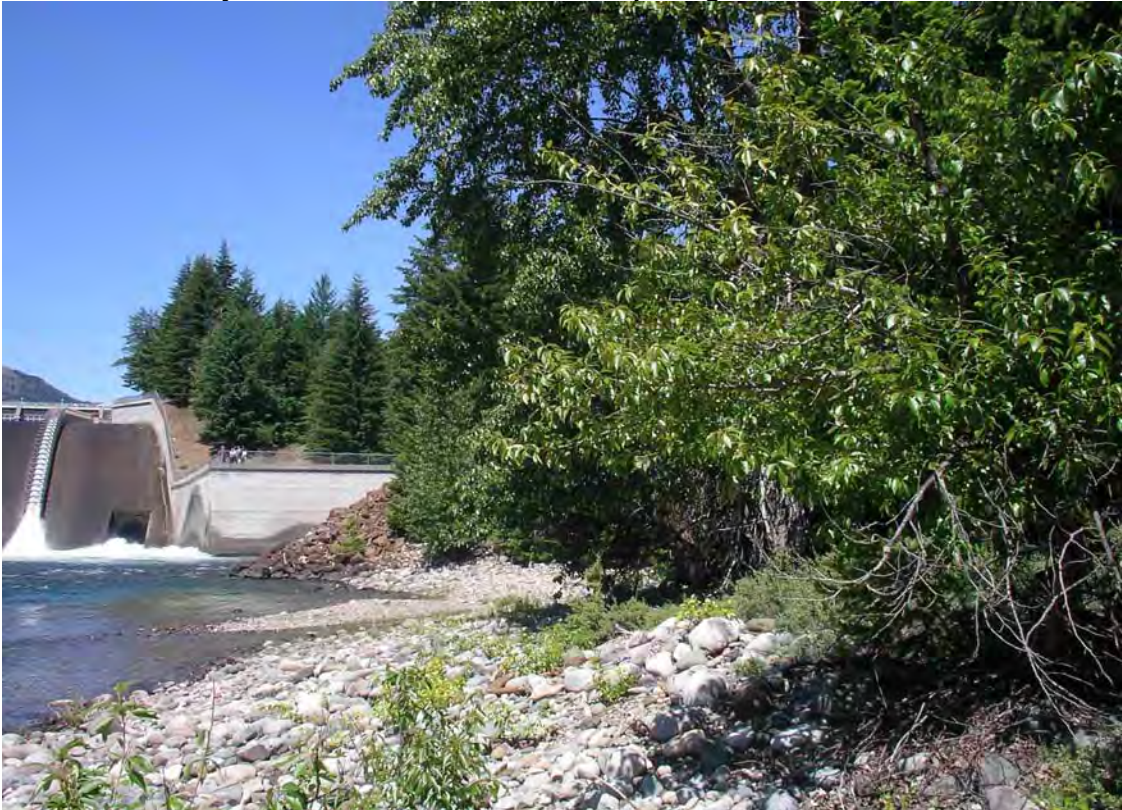
Figure 4-2. Riparian vegetation removed for construction of the adult collection facility. This figure shows the Alternative 2 location of the adult collection facility.
