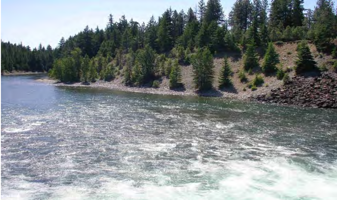
Figure 4-3. Area downstream from Cle Elum Dam where the barrier dam would be constructed for Alternative 2.
