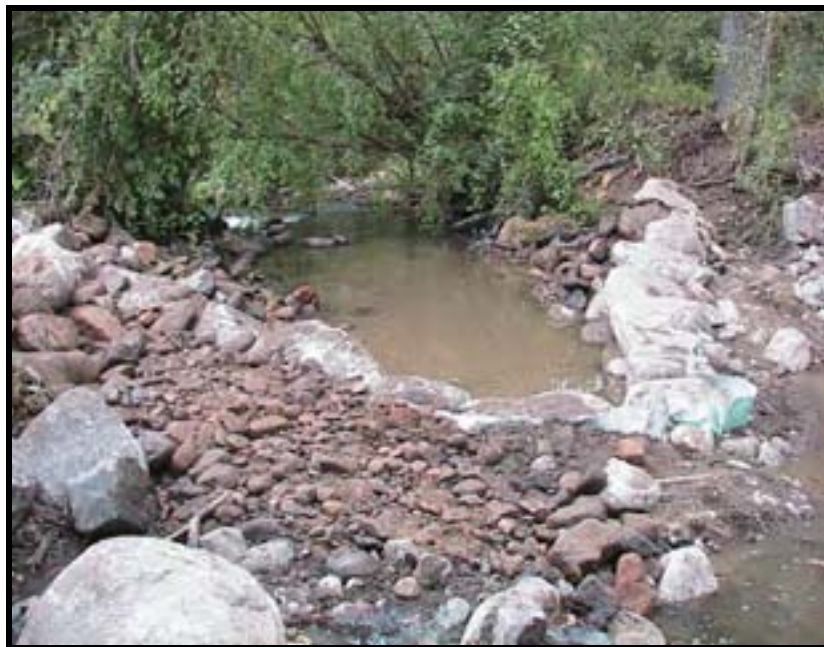
Photo A-22. Looking downstream at Weir No. 3 about 3 hours after Photo A-21 above was taken. The weir has been backfilled and the scour hole excavated.
