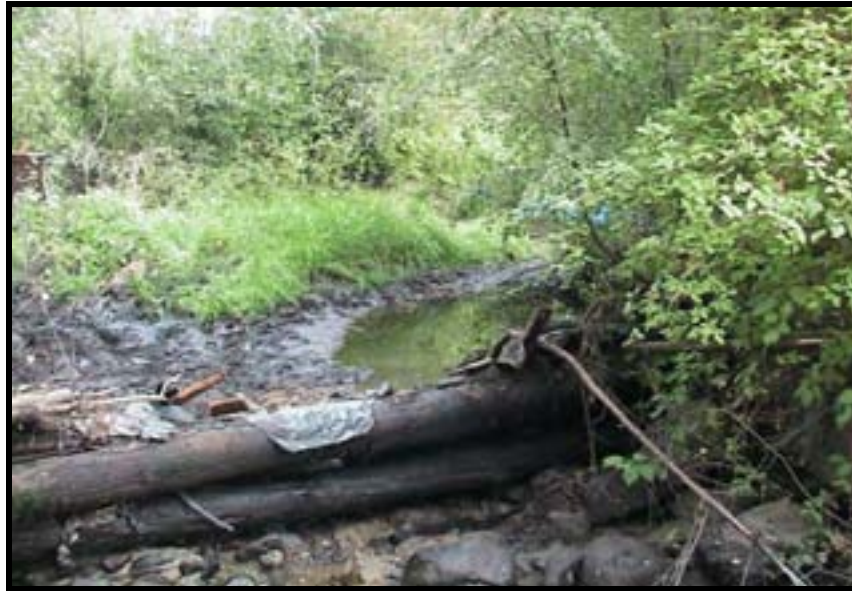
Photo No. 19. The Lower Stokes Diversion Dam was deconstructed in stages to facilitate electro-shocking and removal of fish from project area.
