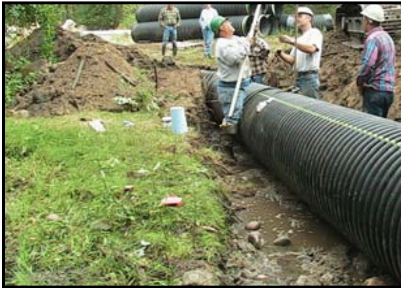
Photo A-5. Excavation crew checking for proper slope of dewatering pipe.
