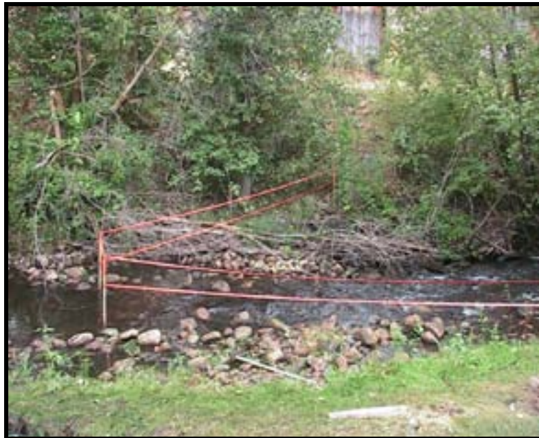
Photo A-2. Preliminary layout of upper weir (Weir No. 1); flow is from left to right.
