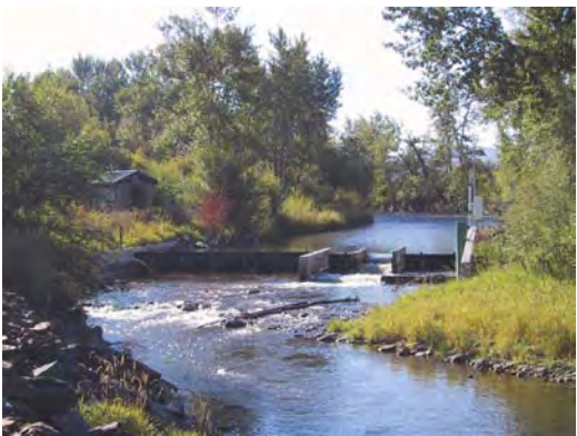
Photo 2.3-1. L6 Diversion structure on the Lemhi River.
