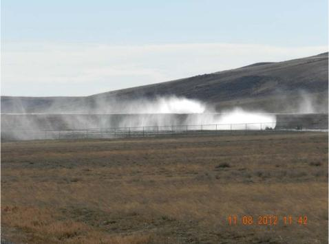
Figure 3. Aerial drift of evaporator spray extends beyond two commercial oilfield wastewater disposal facilities onto adjacent lands, Carbon County Wyoming (Sep 20, 2010 and Nov 8, 2012).
