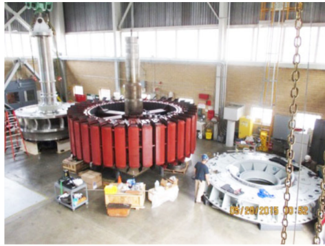
New turbine runner installed for unit 1 (4 percent efficiency gain).
