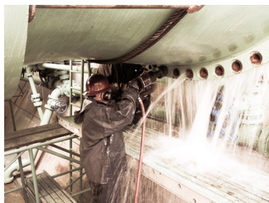
"Unbolting the Penstock" by Joaquin Mancias
