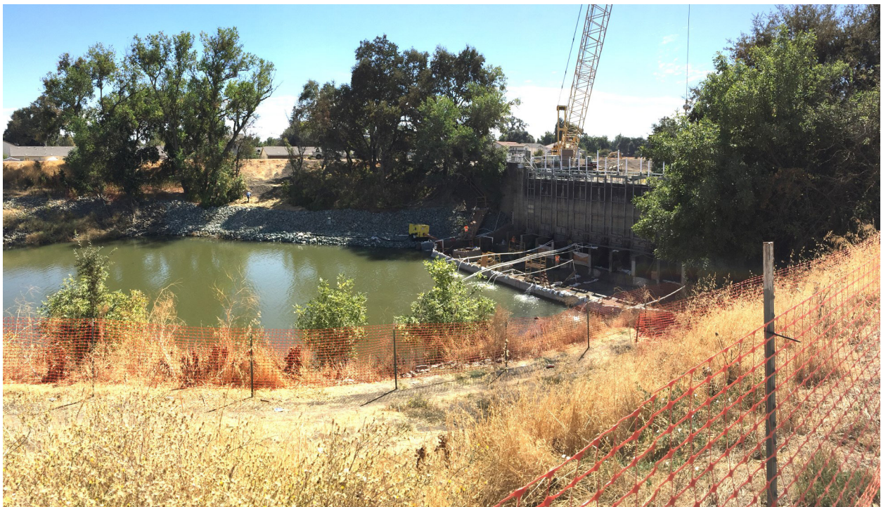
Concrete work in progress at Knights Landing Outfall Gates Project
