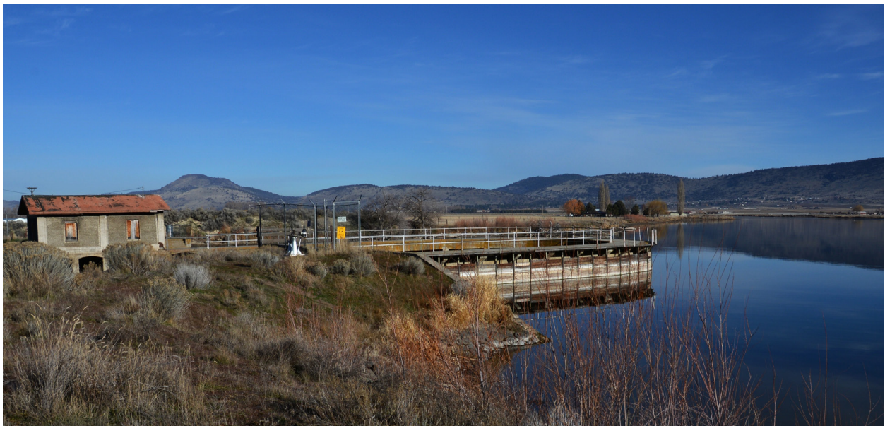
Lost River Diversion Dam, Klamath Project
