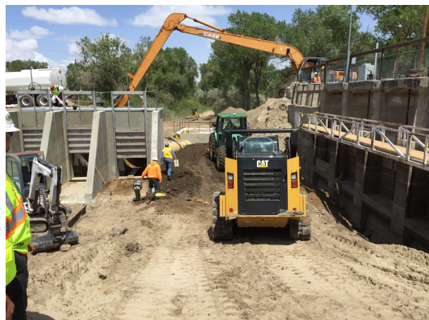
V-Line Canal breach repairs
