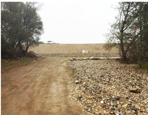
Construction successfully completed in June 2015, reducing the risk of internal erosion due to seepage through the Dike 1 embankment.
