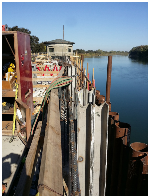
Sacramento River Joint Intake RD 2035 fish screen construction
