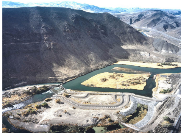
LBAO's Derby Dam services both Newlands and Washoe projects, diverting water down the Truckee Canal to Lahontan Dam
