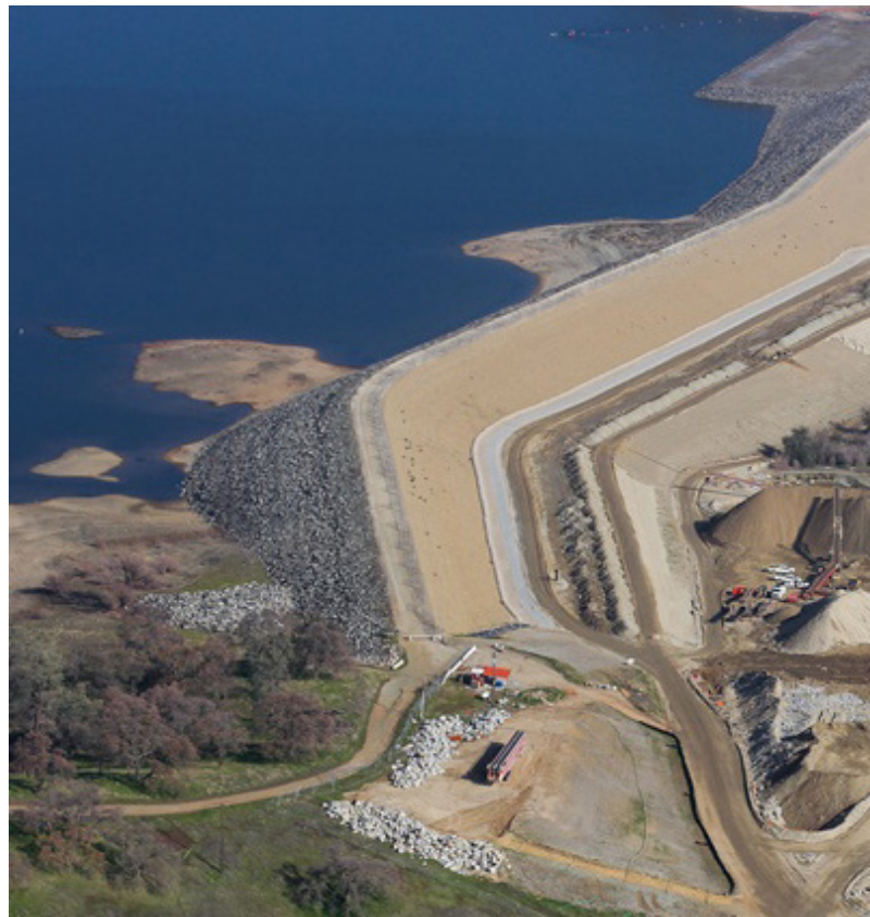
Aerial photograph of Mormon Island Auxiliary Dam during construction
