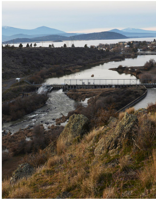
Link River Diversion Dam
