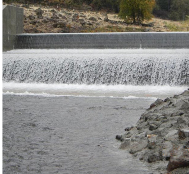
Baldwin Creek Fish Barrier
