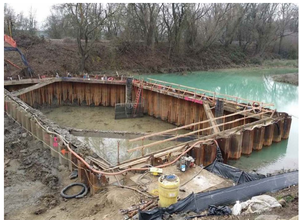
Outlet structure dewatering
