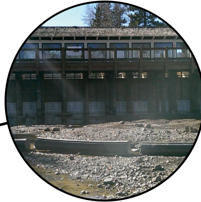
Upgrades of all 17 sluice gates.
