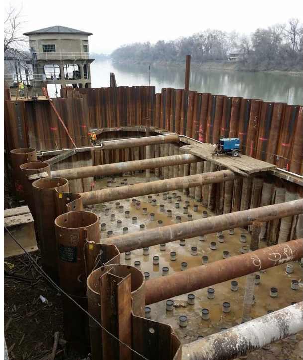
Coffer dam after dewatering
