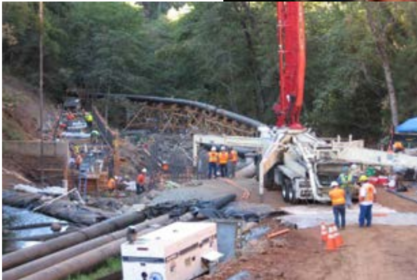
Contractors construct North Battle Creek feeder diversion dam, fish screen and ladder.
