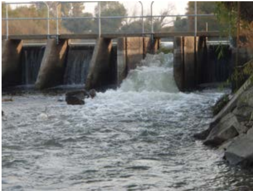
After: Sack Dam and the same fish-ladder structure, as shown on the previous page, but with water flowing through it in 2010.
