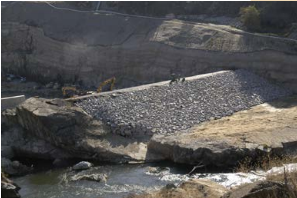
View of a temporary cofferdam nearing completion.
