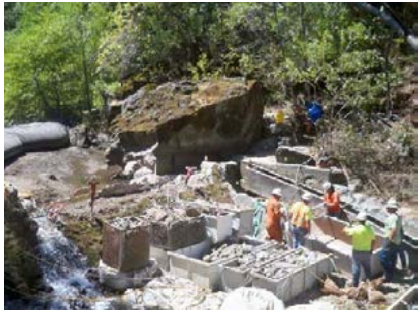
Contractors demolish Wildcat Dam on Battle Creek.
