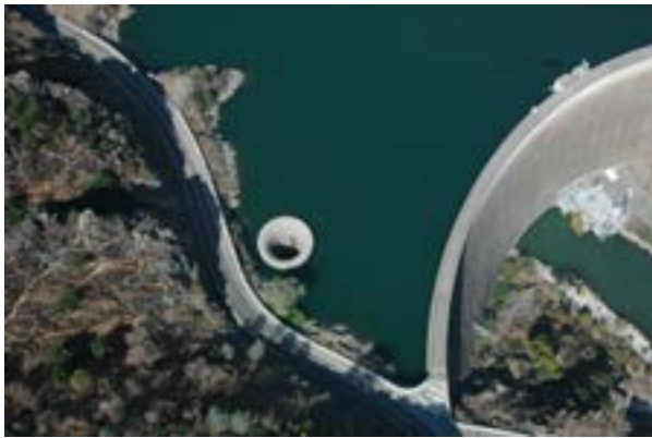
Monticello Dam in the Solano Project is noted for its "glory hole," a type of spillway with an intake shaped like an inverted bell.
