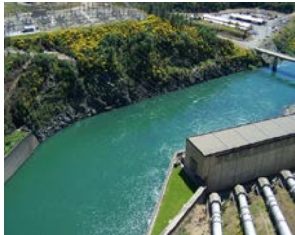
The hydroelectric power plant at Shasta Dam is one of many in the Central Valley Project.
