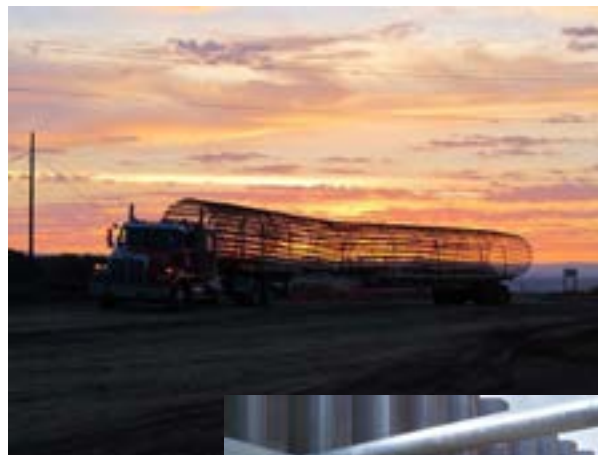
Workers deliver a reinforcement cage for a bridge pier.
