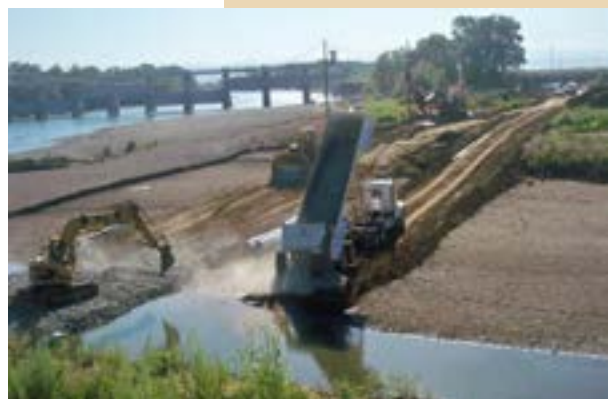
Contractors building an access road.
