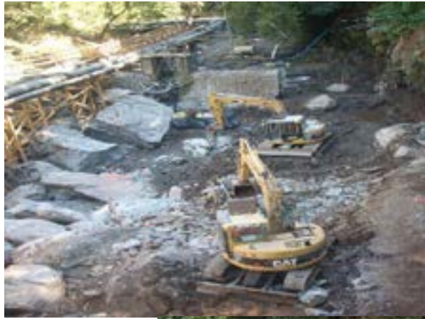
Excavating fish screen and ladder.
