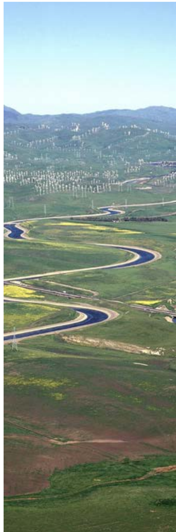
The Delta-Mendota Canal and the California Aqueduct.
