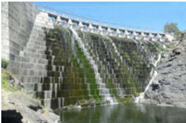
Copco 1 Dam, which is 115 feet in height, is another of the dams that may be removed from the Klamath River.
