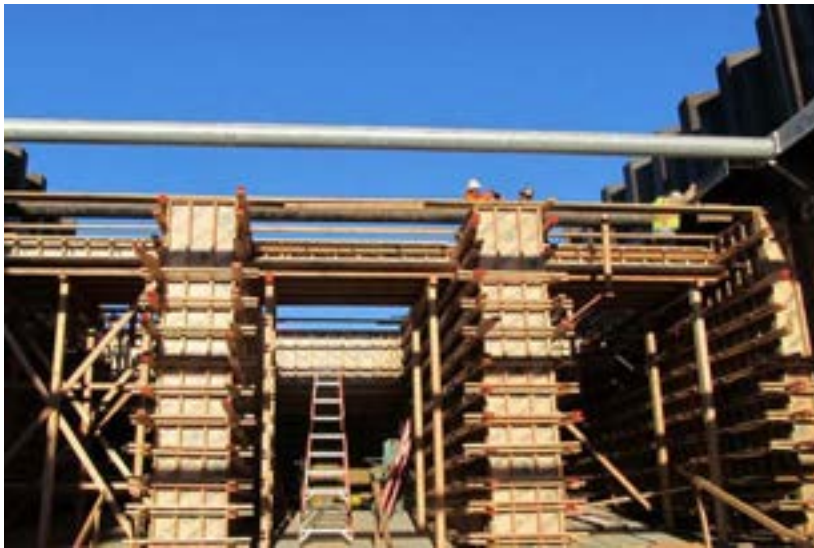
The siphon outlet structure under construction.
