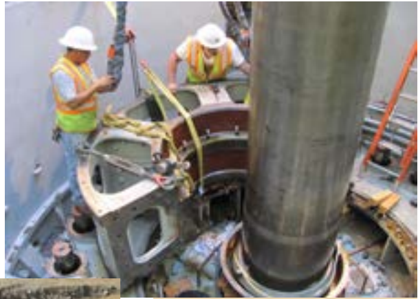
Contractors remove a turbine bearing as part of the hydroelectric plant overhaul.
