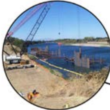
$220 million Project Underway at Red Bluff Diversion Dam
