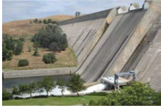
Releases from Friant Dam are being used in restoration of the San Joaquin River.
