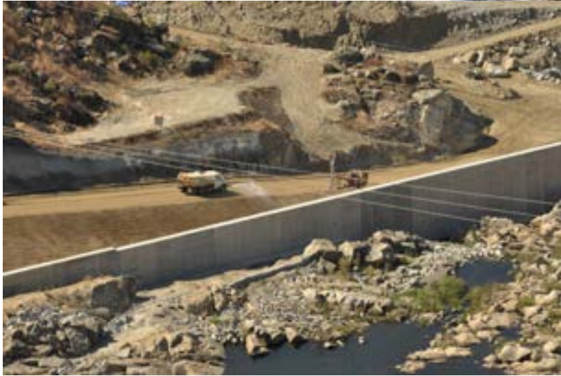
A view of the lower stilling basin access road and cofferdam wall.
