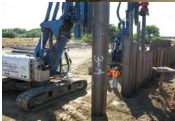
Diesel hammers drive sheet piles.
