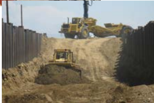
Heavy equipment excavates the canal on the east side of Red Bank Creek.
