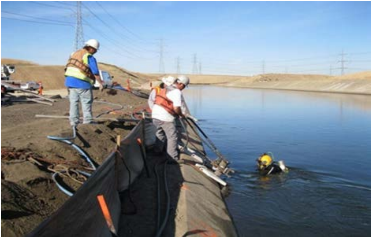
Diver begins cutting canal's concrete liner in the first stages of the project.
