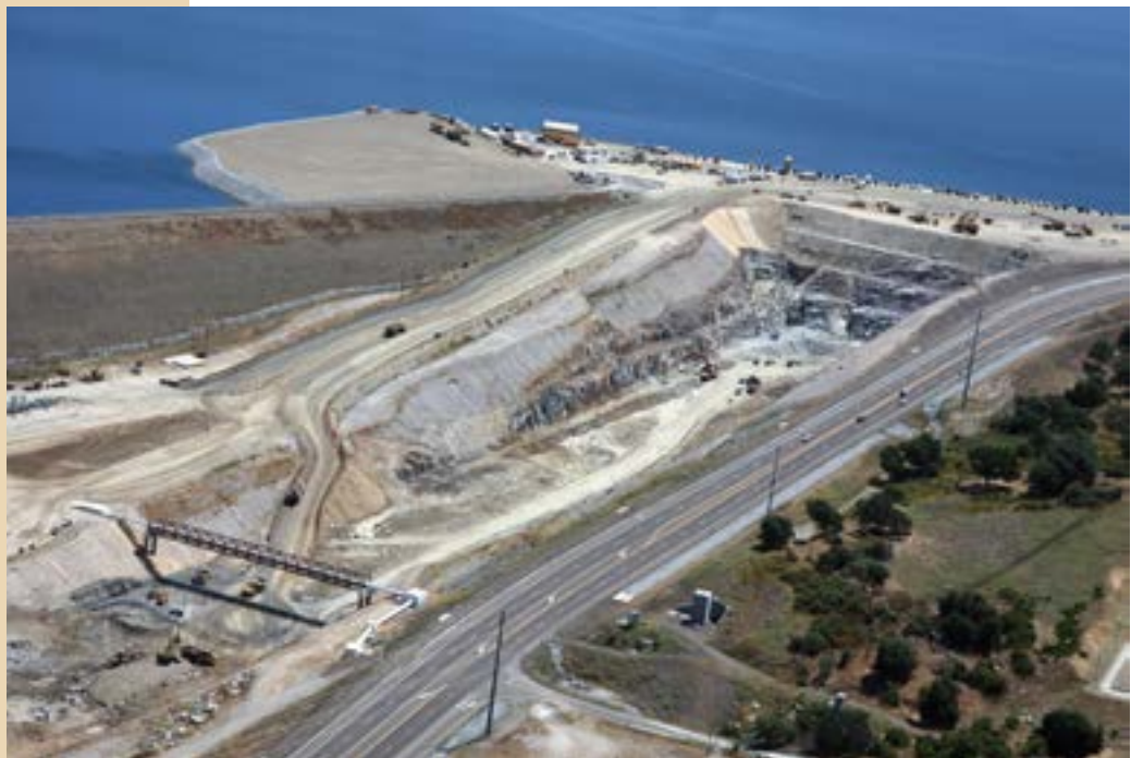
View of upper auxiliary spillway, expanded overlook area, and Natoma pipeline bridge in the foreground.
