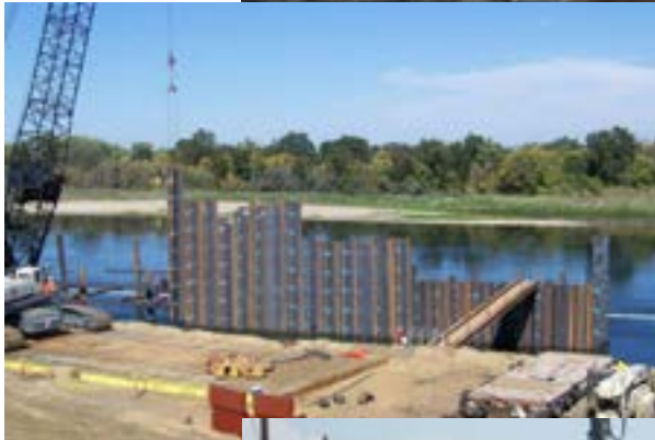
Installing coffer dam sheet piling for fish screen.
