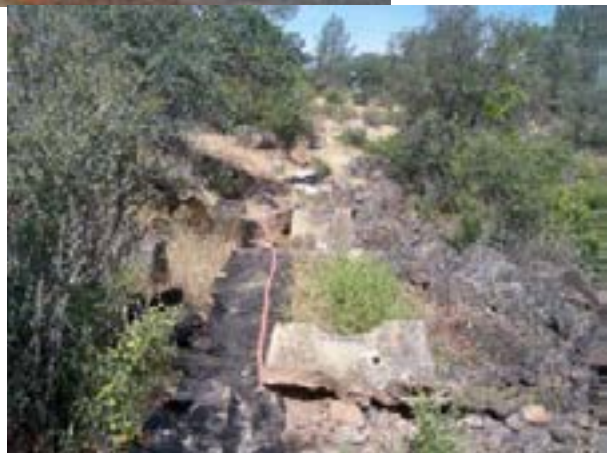
The concrete footings for the pipeline.
