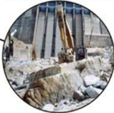
Increasing Safety at Major Reservoir
