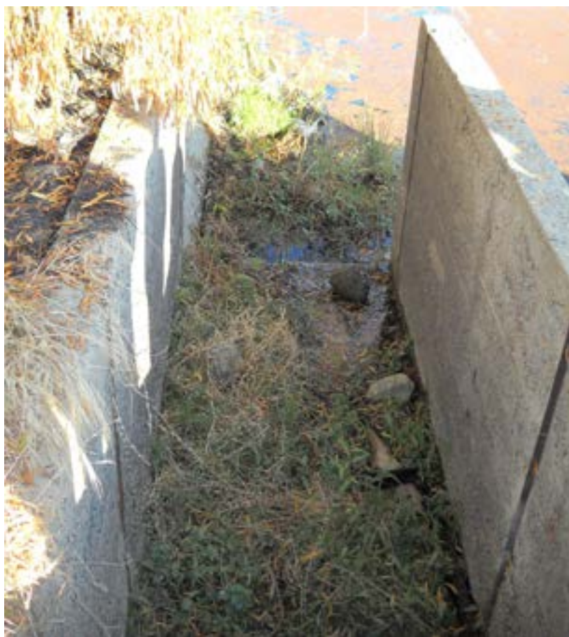
Before: The fish-ladder structure at Sack Dam on the San Joaquin River in 2009 before the return of flows.
