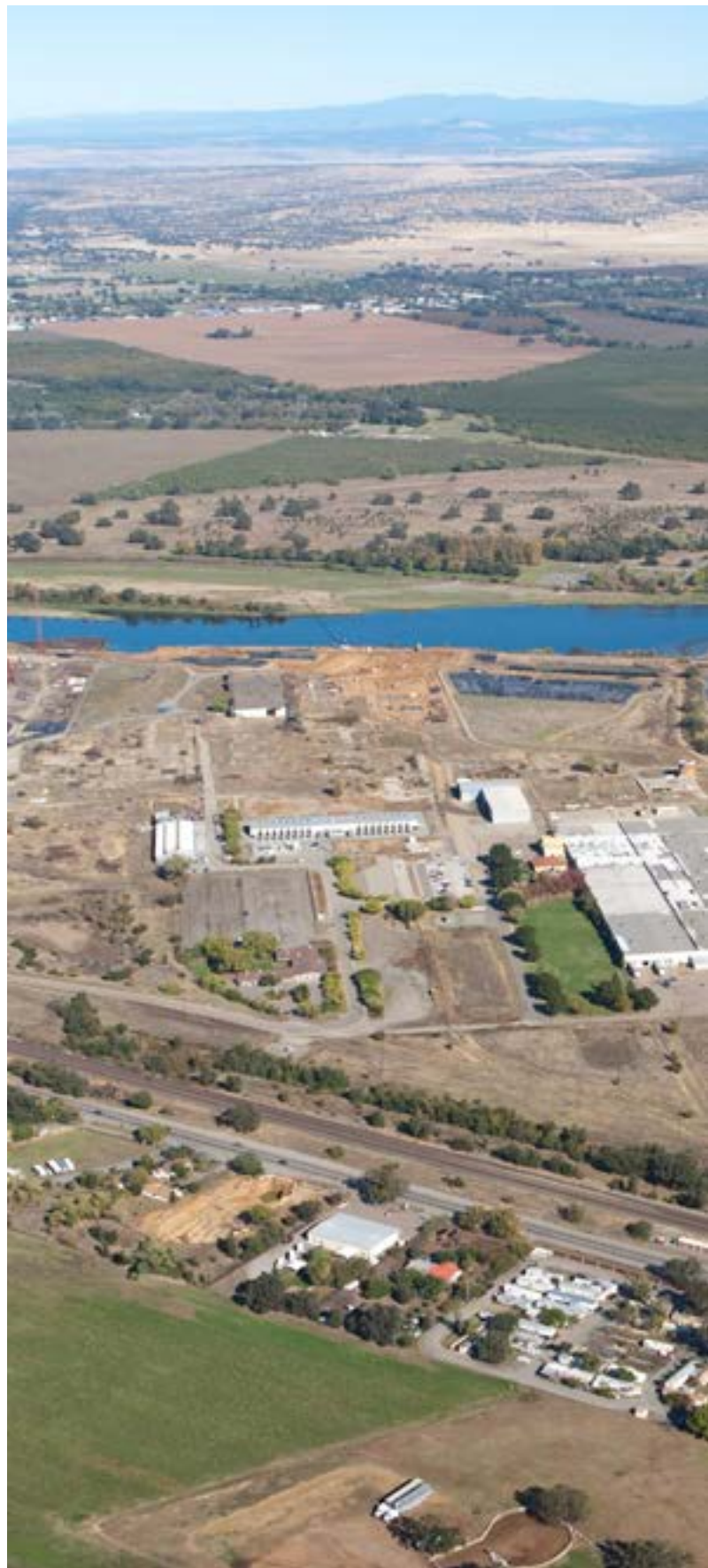
Red Bluff Diversion Dam is shown in upper right corner.
