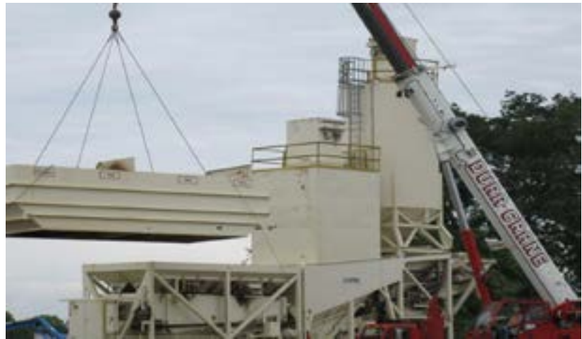
Workers assemble portable concrete mixing plant for onsite production.
