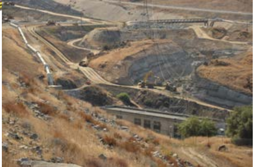
Contractors build an access road to the new auxiliary spillway, with a new pipeline shown at left.
