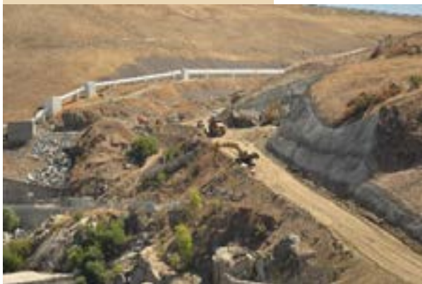
Construction improvements underway at Folsom Dam.
