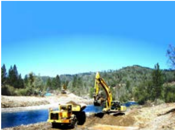
Contractors work on restoration of Trinity River.
