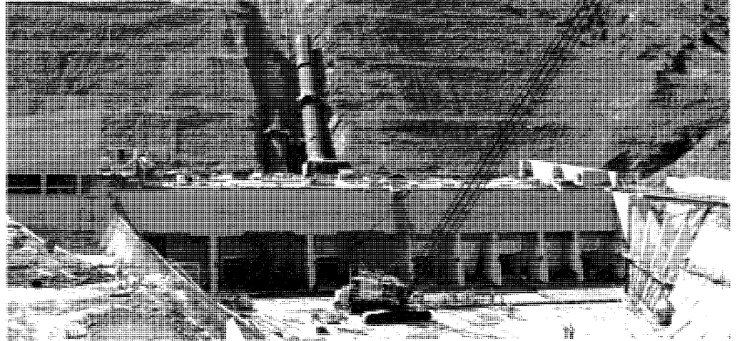
Ongoing construction at Havasu Pumping Plant.
