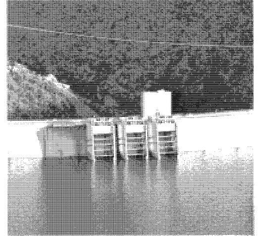
Three selective withdrawal structures.
