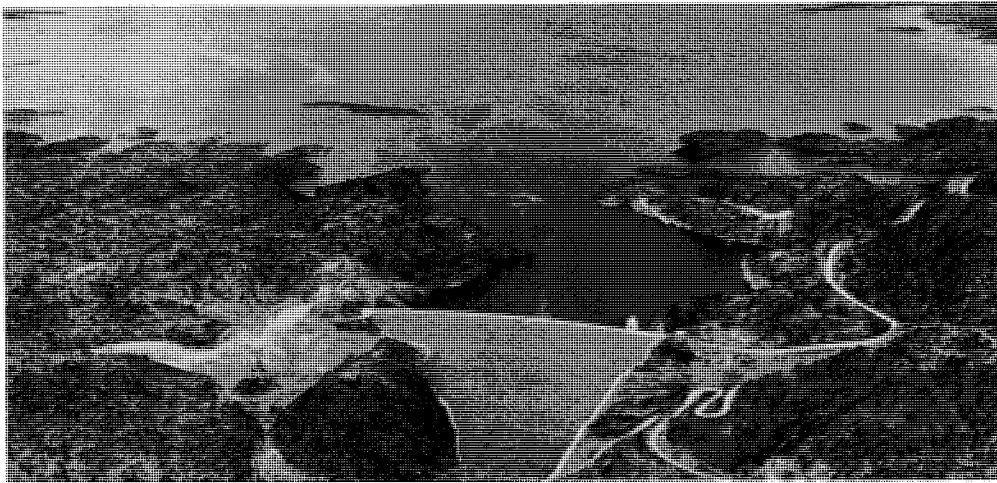
Alamo Dam and Lake
