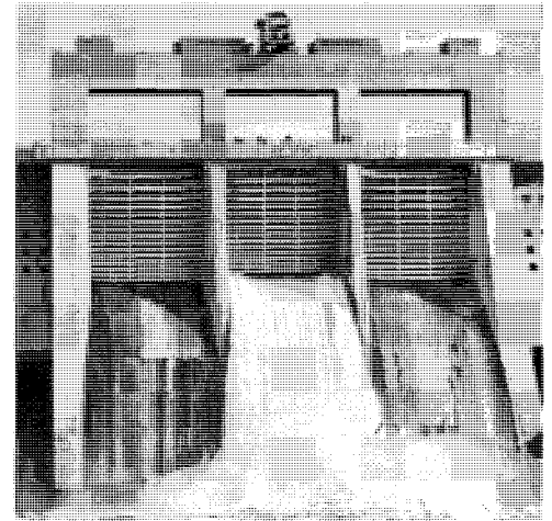
Davis Dam spillway gates
