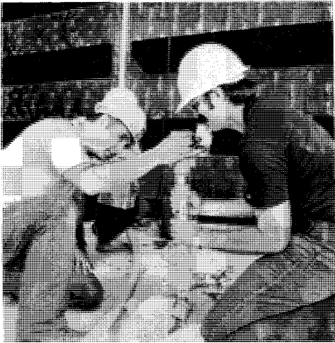
Workers at Parker Dam
