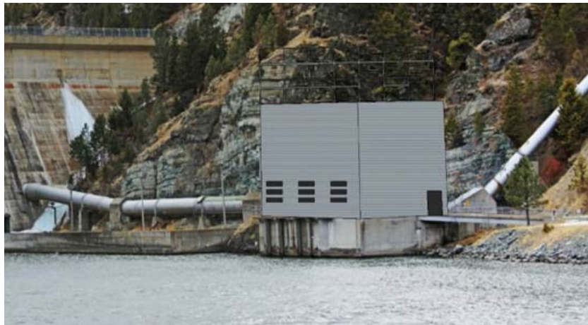
Figure 4. Future Pumping Plant Building Enclosure.
